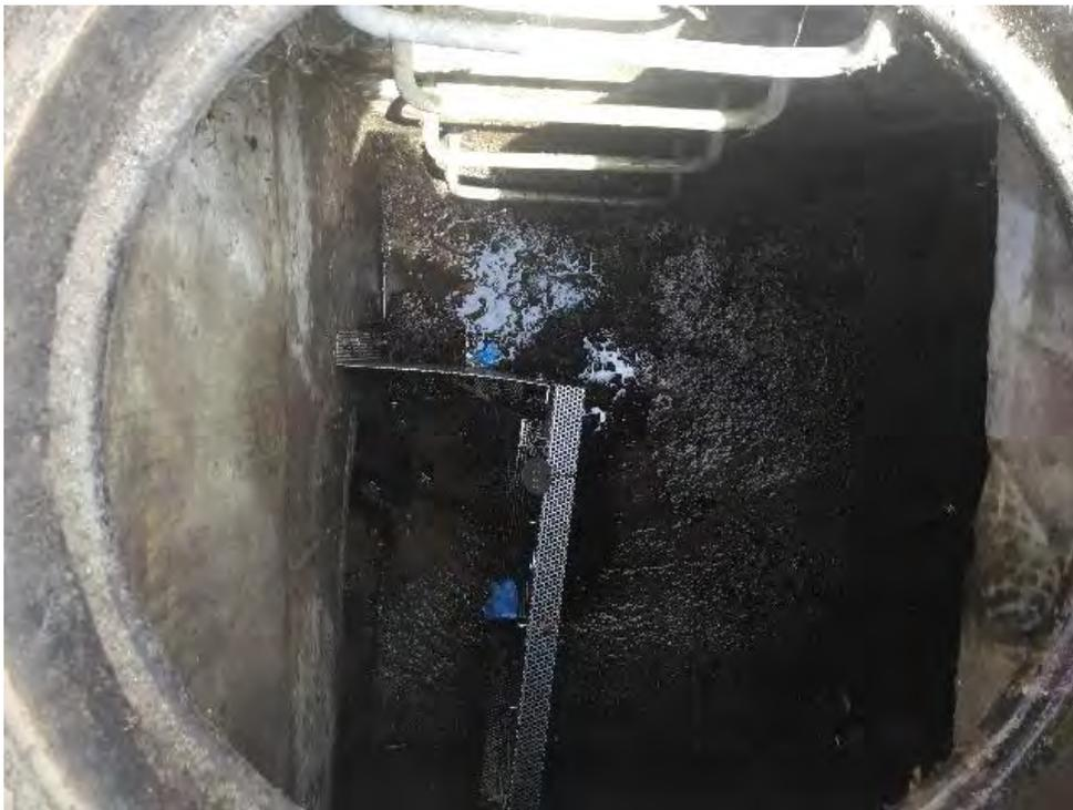
**Figure 2: Cleaned catch basin (County of Ventura catch basin)**
