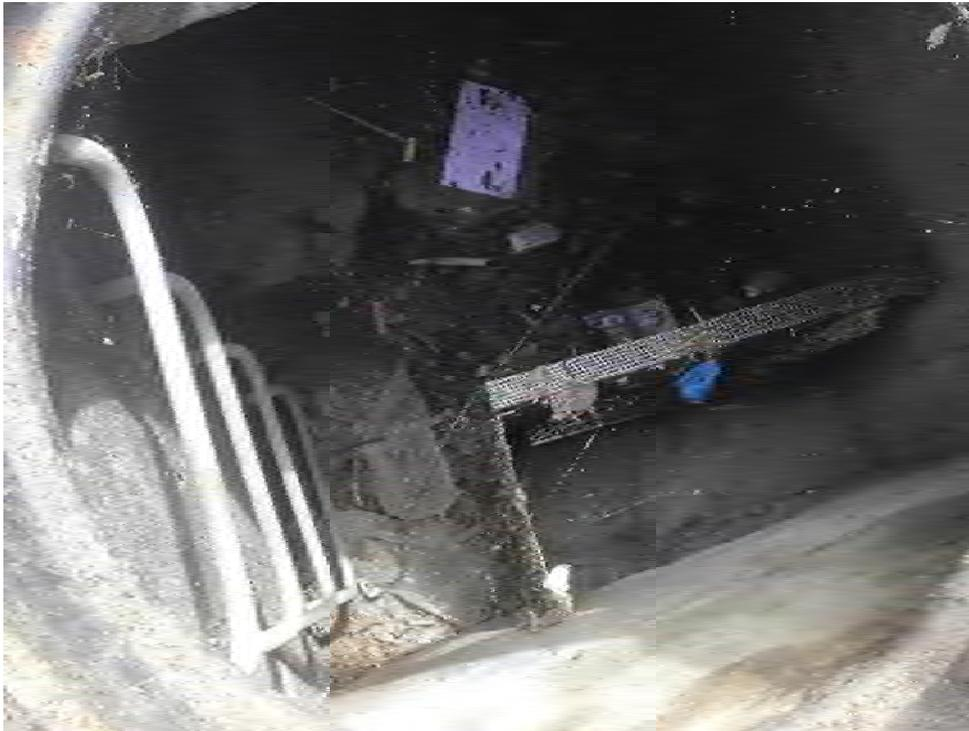
**Figure 1: Catch basin prior to cleaning (County of Ventura catch basin)**
