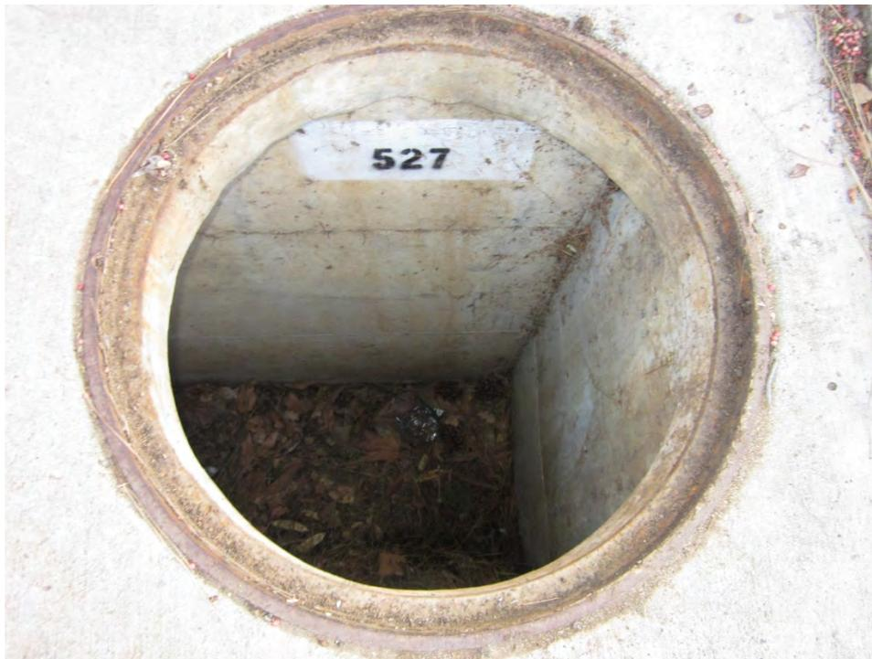
**Figure 1: Catch basin prior to cleaning**
