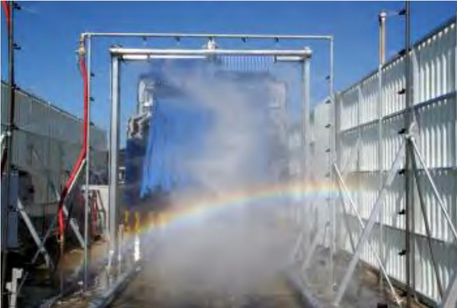
The Permittees have been successful in implementing applicable BMPs to eliminate wash water discharges from vehicles and equipment washing. As municipal facilities are constructed, redeveloped, or replaced all vehicle wash areas will be plumbed to the sanitary sewer or be self-contained with all wastewater disposed of legally.
