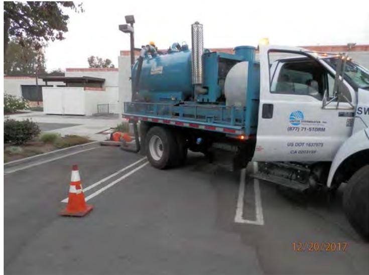
*Catch Basin Cleaning Using a Vacuum Truck*
