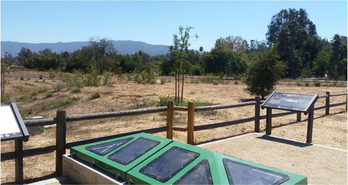
3. El Rio Retrofit for Groundwater Recharge. Construction was completed in March 2016. The project captures 100% nuisance flows and the first flush stormwater discharges from 46 acres of residential community of El Rio for infiltration and groundwater recharge. Total project cost is \$1.3M.
