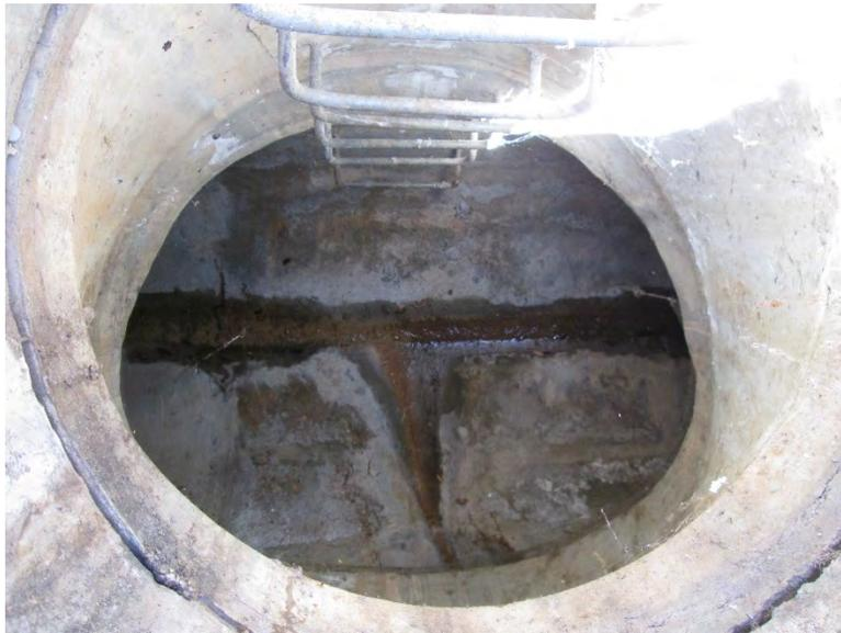
A photograph looking down into a storm drain manhole. The manhole is circular and made of concrete. A metal grate is visible at the top. A trickle of water is flowing down the center of the drain. The interior of the manhole shows some sediment and debris.                                       |
