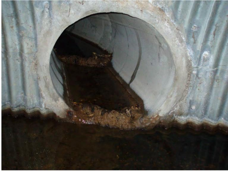
A photograph showing a pipe's outfall submerged in a pond. The pipe is made of corrugated metal and is surrounded by a concrete structure. The water level is high, and the pipe's interior is visible, showing some debris and a dark, stagnant water surface.                          |
