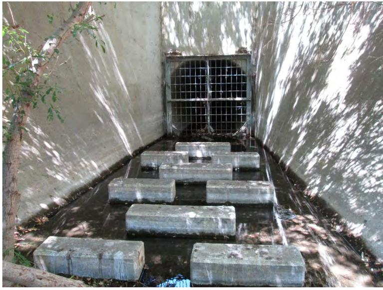
A photograph showing a storm drain outfall in a narrow alleyway. The drain is a concrete channel with several large concrete blocks placed across it to create a series of steps or a barrier. The alleyway is flanked by concrete walls, and there are shadows cast by trees and foliage on the walls. |
