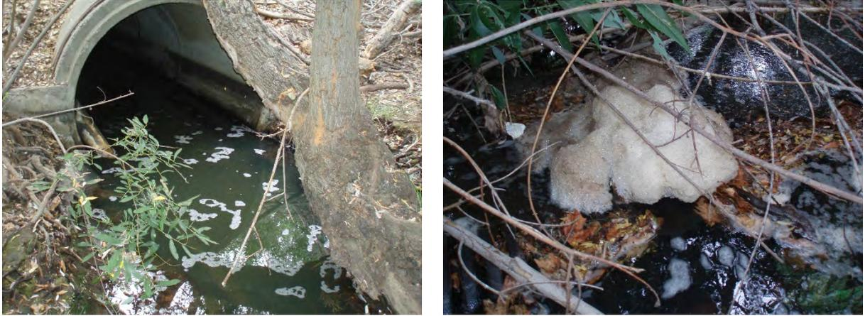
**Fig. 2.3. Storm drain outfall with temporary high flow outputs (left) and resulting foam in creek downstream (right)**
