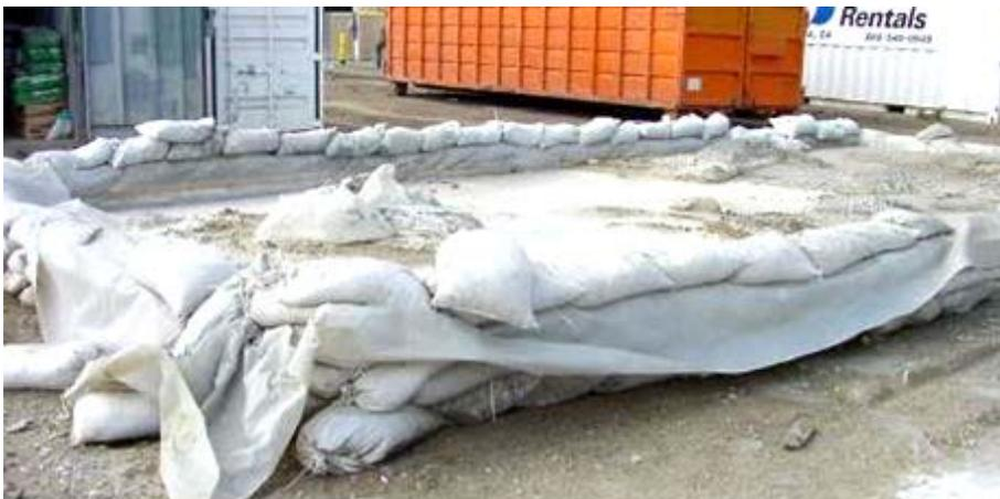
*Concrete washout at construction site*
