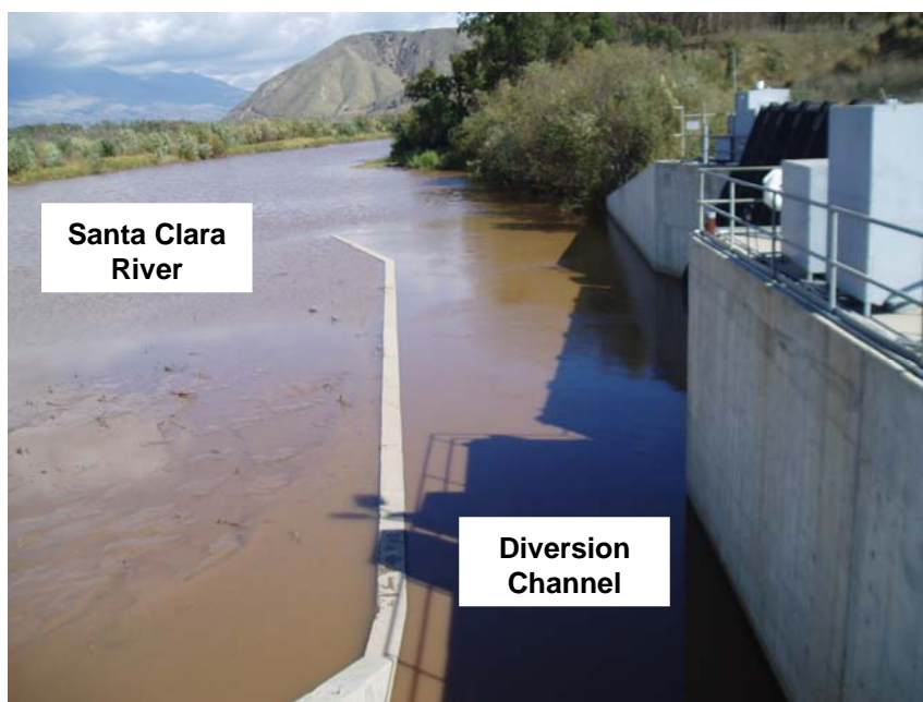
Figure 10: ME-SCR Freeman Diversion Dam (Facing Upstream)
