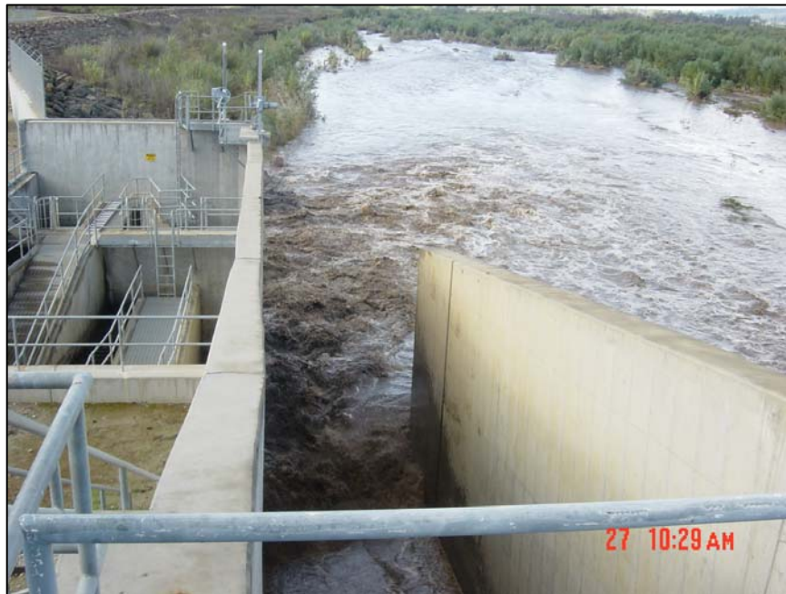
Figure 12: River Diversion Gate (Facing Downstream)
