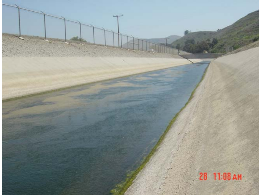
Figure 13: Infiltration Channel (Facing Upstream)
