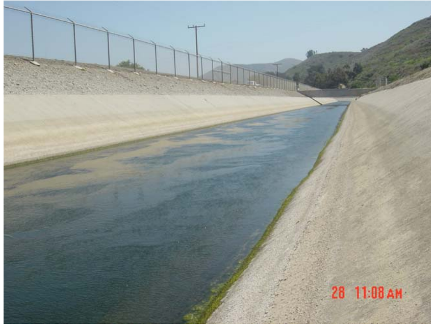
Figure 13: Infiltration Channel (Facing Upstream)
