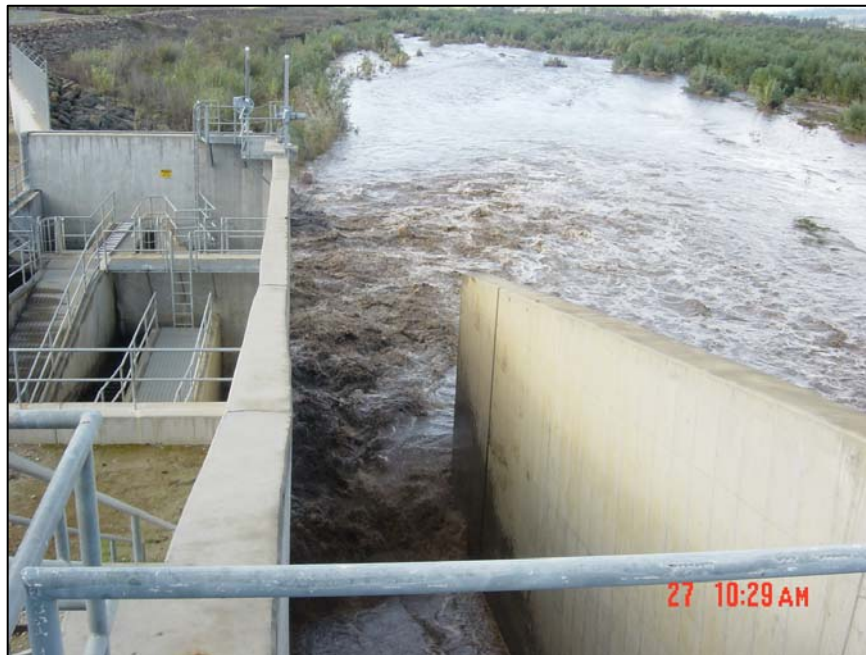
Figure 12: River Diversion Gate (Facing Downstream)
