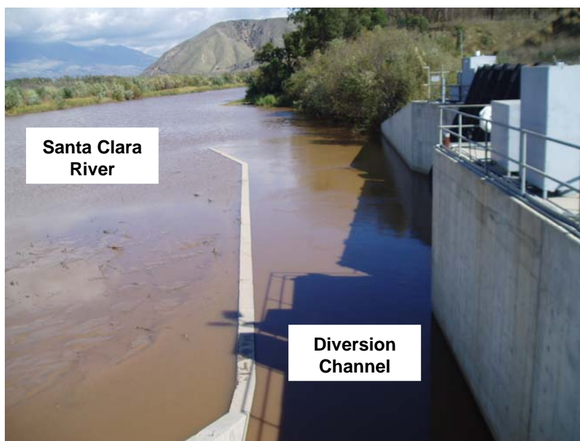
Figure 10: ME-SCR Freeman Diversion Dam (Facing Upstream)
