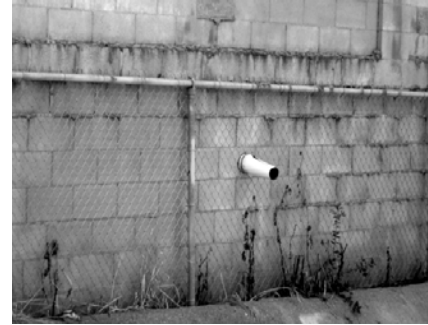
Example of an Illegal Connection
