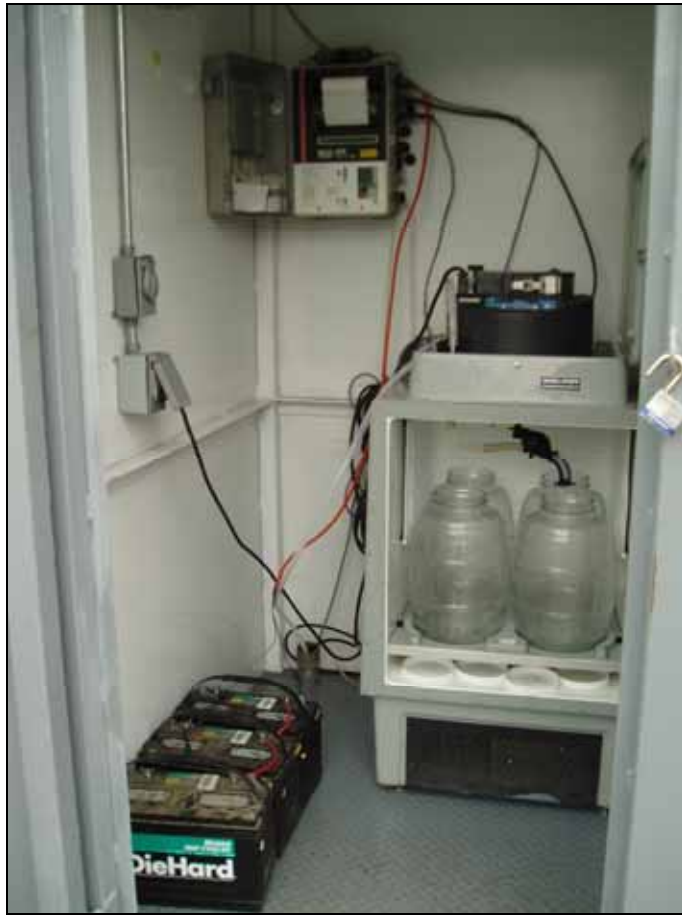
Figure 1: ISCO 6712 refrigerated sampler, ISCO 4230 flowmeter, and steel enclosure at Mass Emission site ME-VR2
