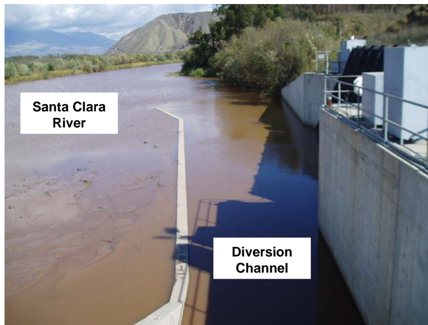
Figure 10: ME-SCR Freeman Diversion Dam (Facing Upstream)
