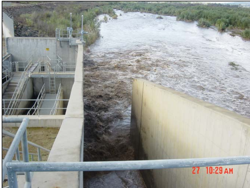
Figure 12: River Diversion Gate (Facing Downstream)
