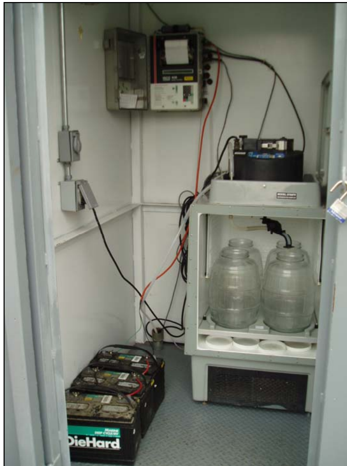
Figure 3: ISCO 6712 refrigerated sampler, ISCO 4230 flowmeter, and steel enclosure at Mass Emission site ME-VR2
