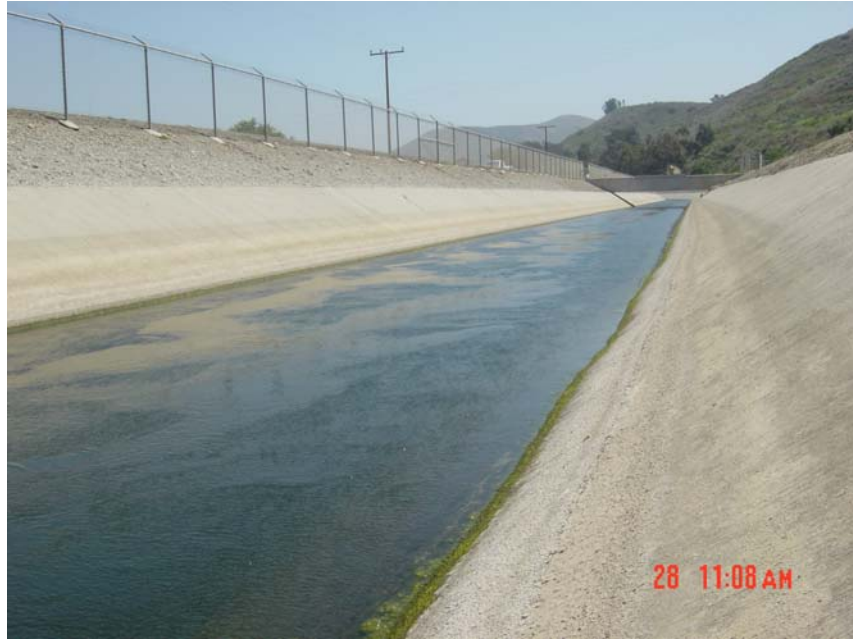
Figure 13: Infiltration Channel (Facing Upstream)
