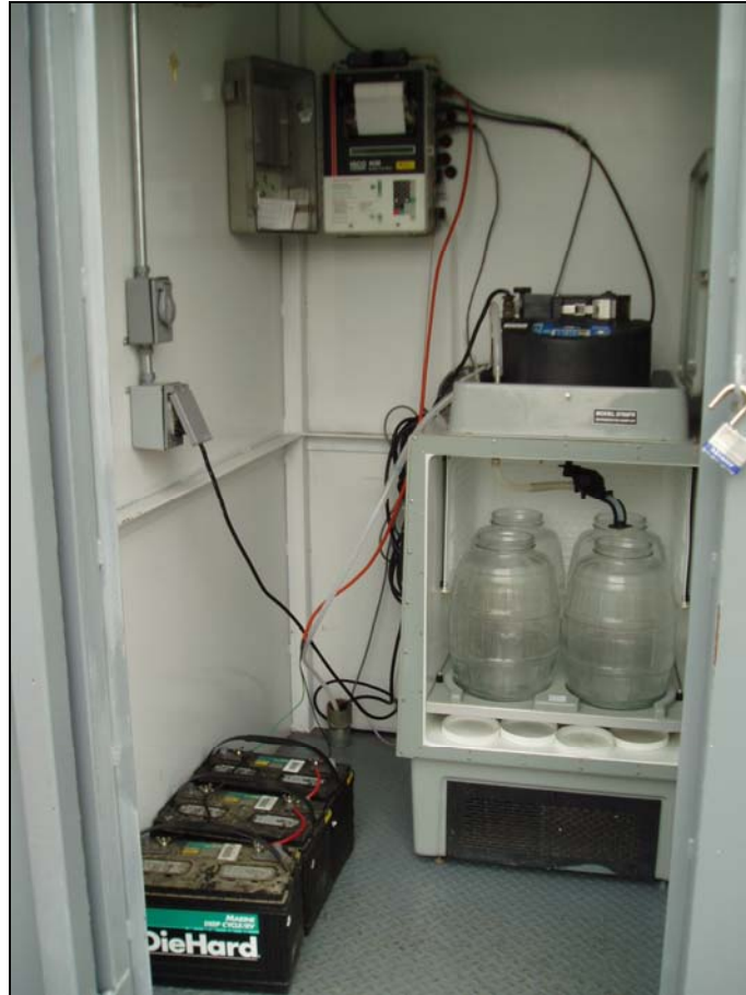
Figure 8: ISCO 6712 refrigerated sampler, ISCO 4230 flowmeter, and steel enclosure at Mass Emission site ME-VR2
