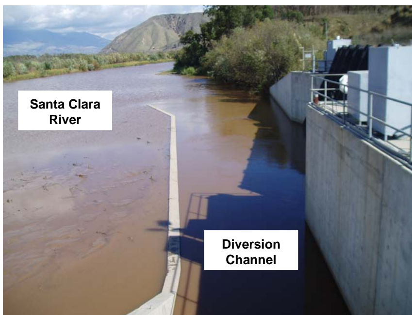
Figure 16: ME-SCR Freeman Diversion Dam (Facing Upstream)
