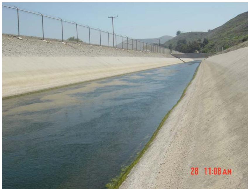
Figure 19: Infiltration Channel (Facing Upstream)
