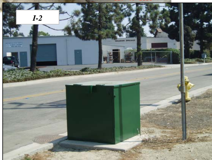
Figure 5: Land Use Station Photos: R-1 (Swan Street) and I-2 (Ortega Street)
