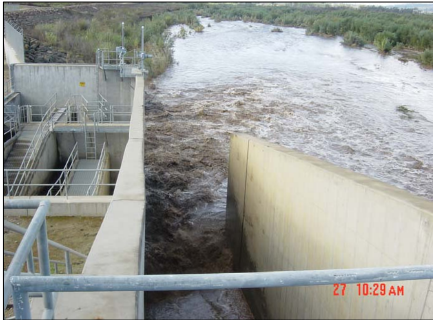
Figure 18: River Diversion Gate (Facing Downstream)
