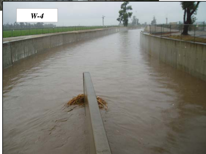
Figure 6: Land Use and Receiving Water Station Photos: A-1 (Wood Road), W-3 (La Vista), and W-4 (Revolon Slough)
