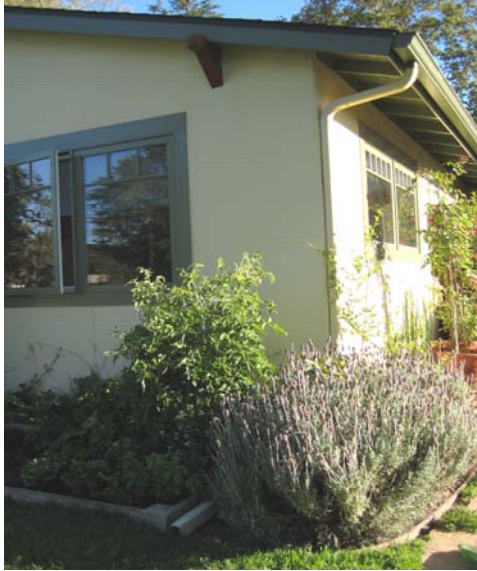
Diverted Roof Runoff City of Santa Barbara
