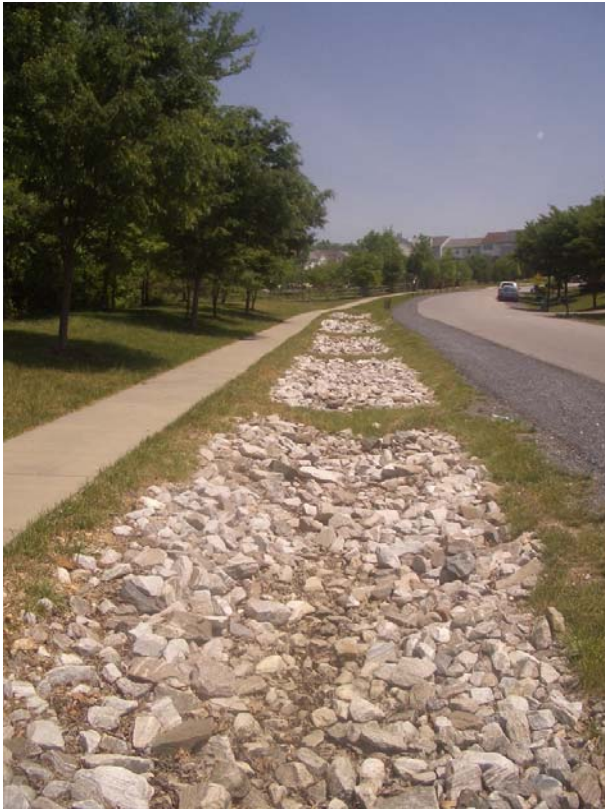
Infiltration Trench
