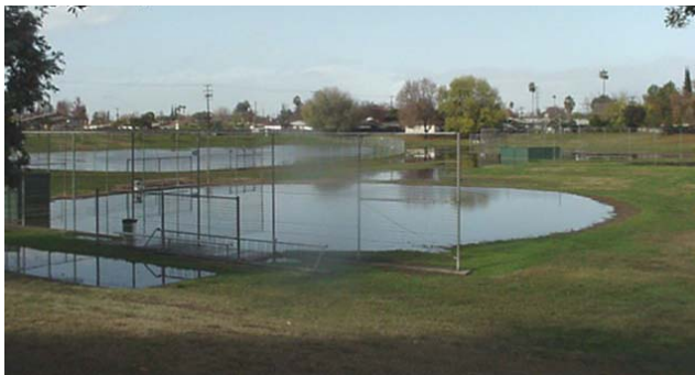
Infiltration Basin in a Fresno, CA Park, Before and After a Rain Event
