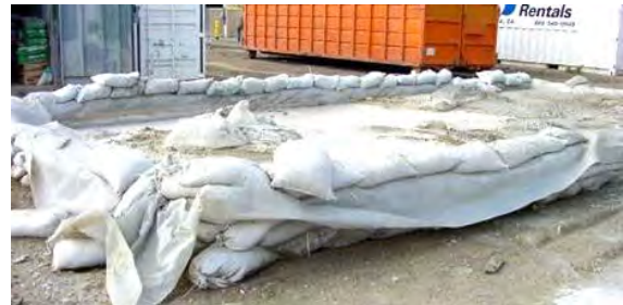
Concrete washout at construction site
