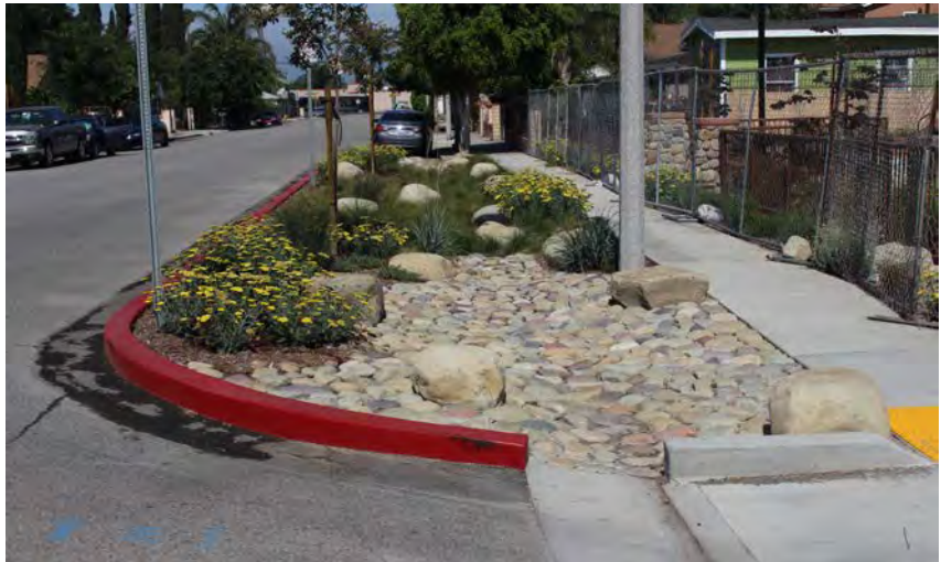
Low Impact Development infiltration BMP
