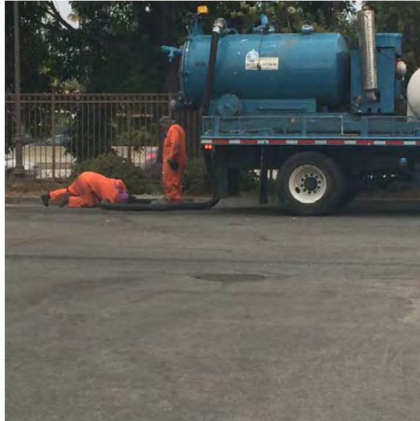
Catch Basin Cleaning Using a Vacuum Truck
