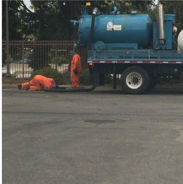
*Catch Basin Cleaning Using a Vacuum Truck*
