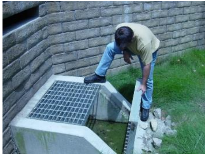
Post-Construction BMP inspection
