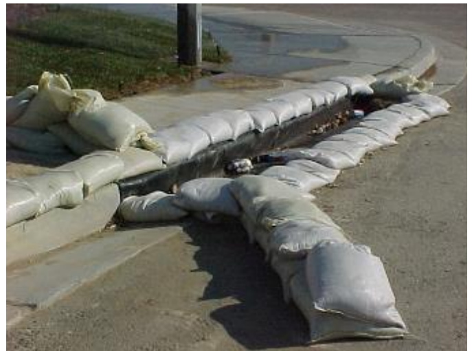
Catch basin protection
