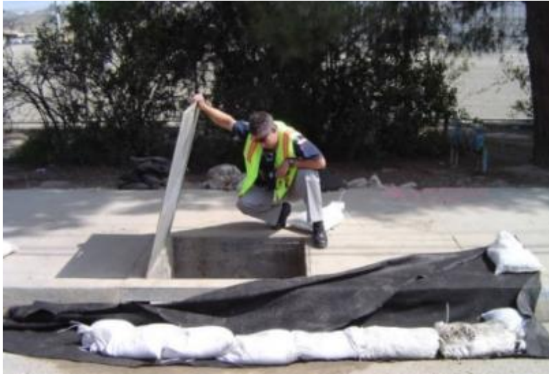
Inspection of catch basin BMPs
