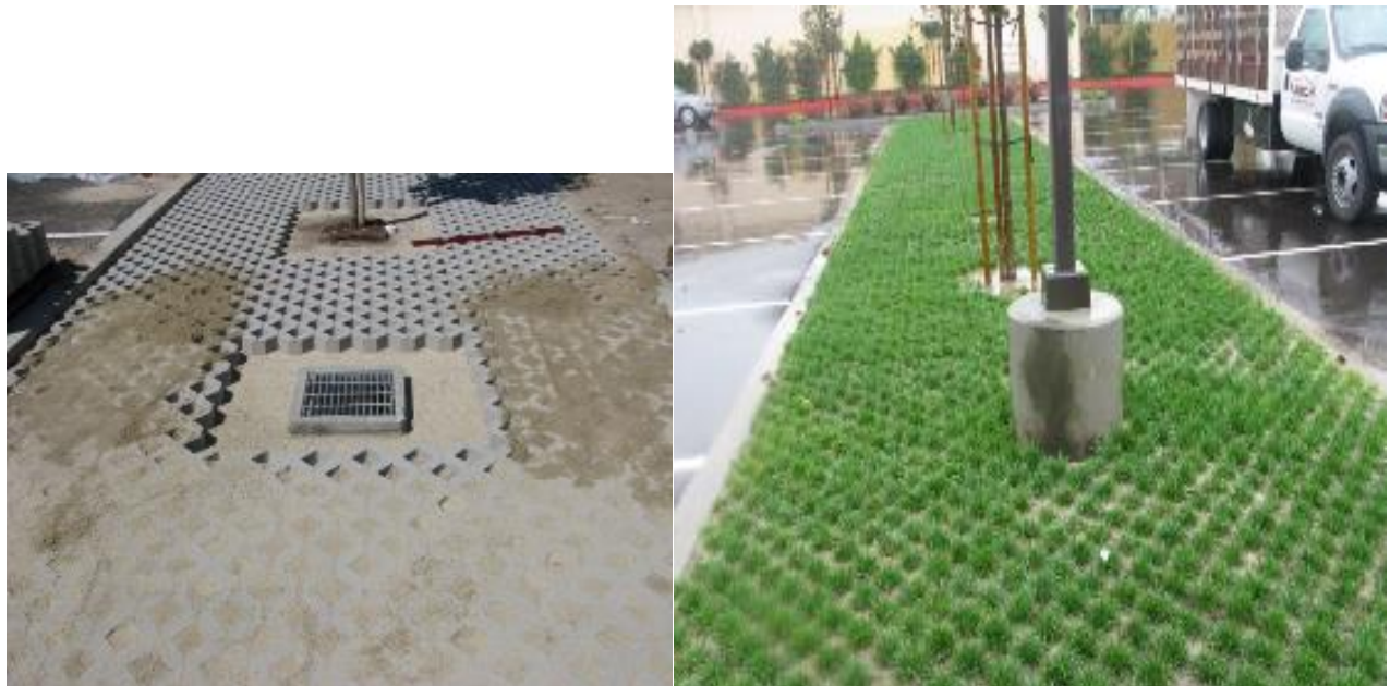
Before and after pictures of infiltration area of parking lot during construction.
