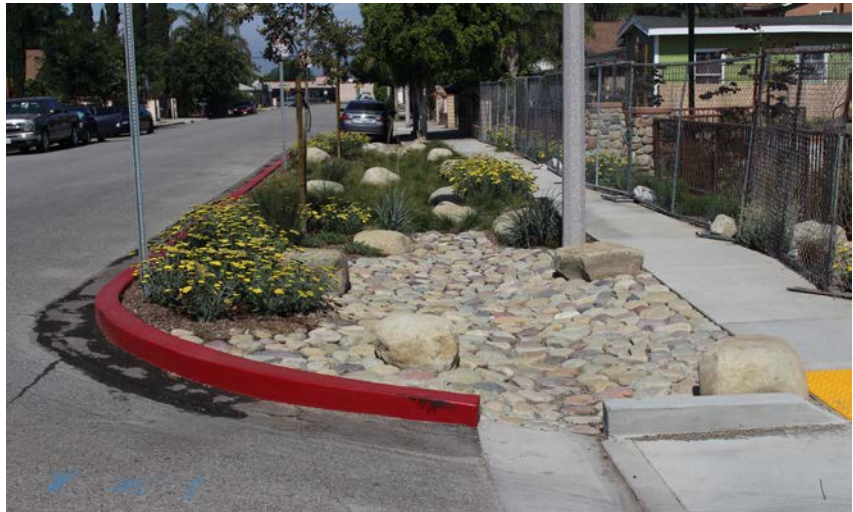
Low Impact Development infiltration BMP
