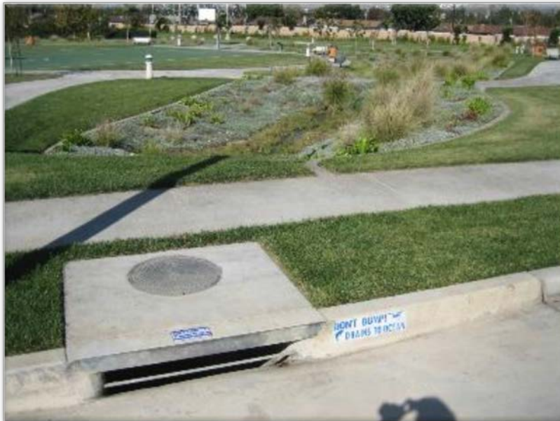
Low Impact Development BMP
