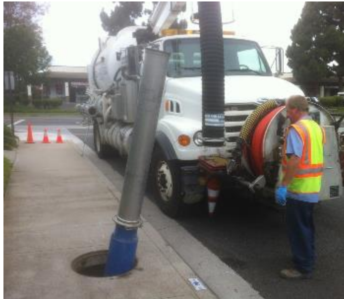
Catch Basin Cleaning Using a Vacuum Truck
