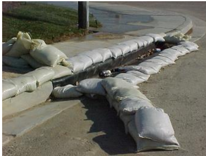
Catch basin protection
