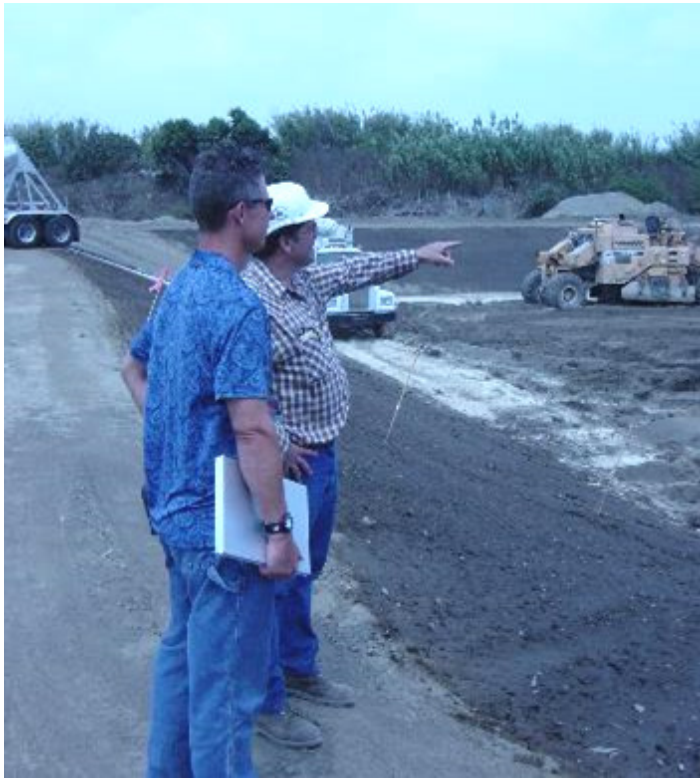
Stormwater inspection at construction site
