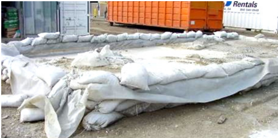
Concrete washout at construction site
