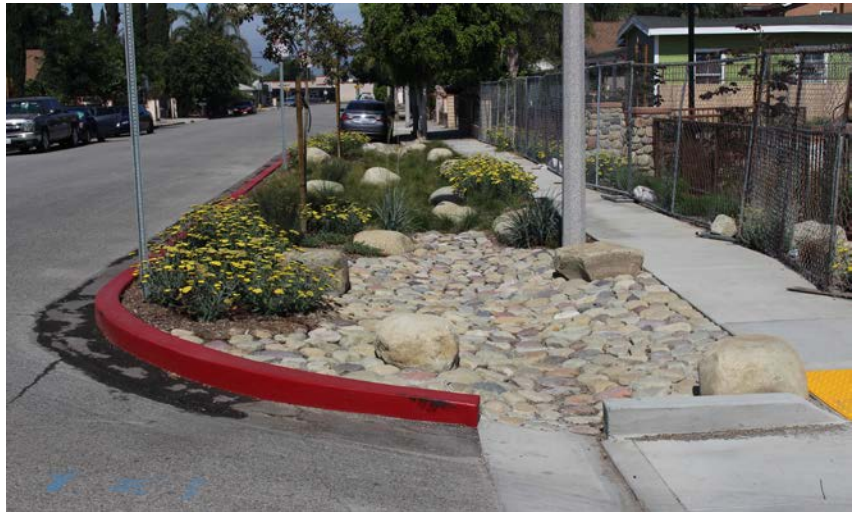
Low Impact Development infiltration BMP
