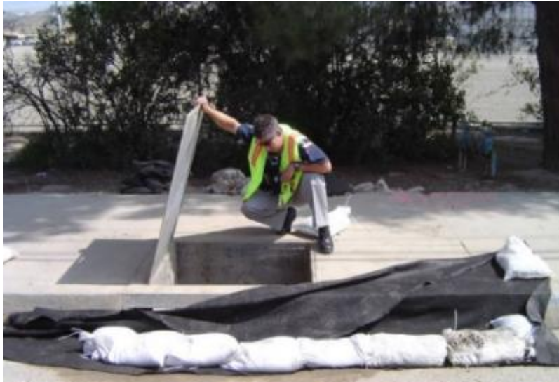
Inspection of catch basin BMPs
