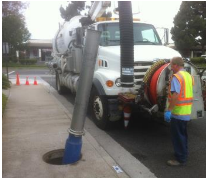
Catch Basin Cleaning Using a Vacuum Truck
