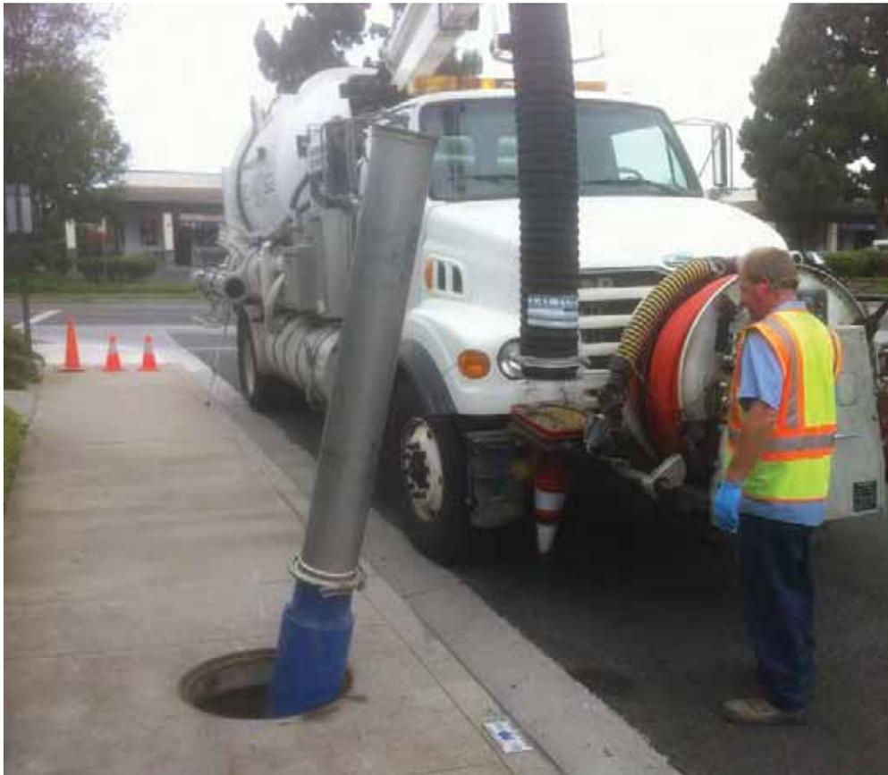
**Catch Basin Cleaning Using a Vacuum Truck**
