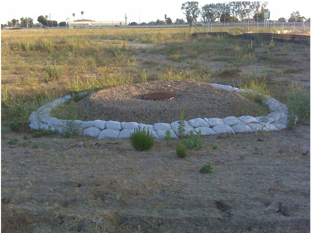
Storm drain protection during construction
