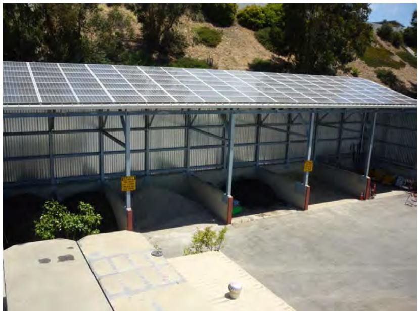
Material storage covers in Camarillo also support solar panels
