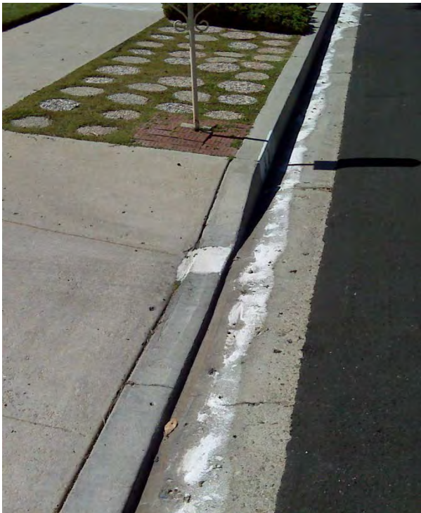
Evidence of an illicit discharge
