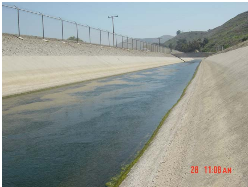
Figure 17: Infiltration Channel (Facing Upstream)
