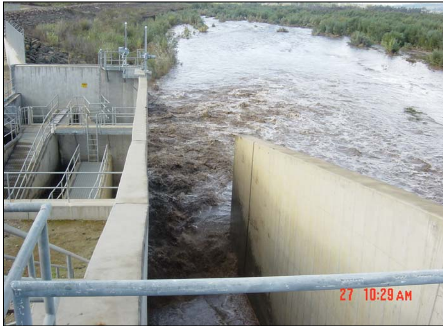
Figure 16: River Diversion Gate (Facing Downstream)
