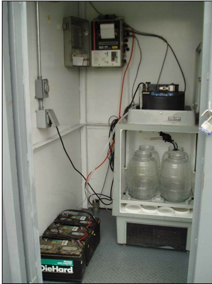
Figure 6: ISCO 6712 refrigerated sampler, ISCO 4230 flowmeter, and steel enclosure at Mass Emission site ME-VR2
