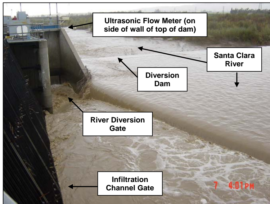
Figure 15: ME-SCR Freeman Diversion Dam (Facing Downstream)
