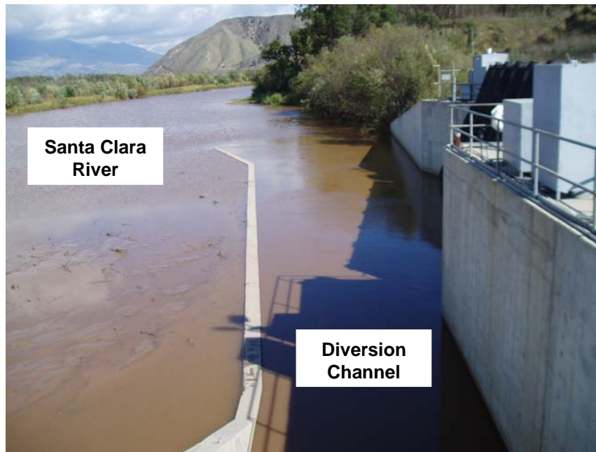
Figure 14: ME-SCR Freeman Diversion Dam (Facing Upstream)
