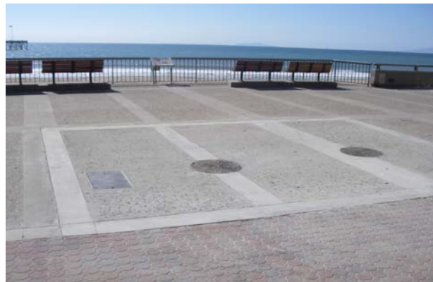
The same site after construction was completed.
