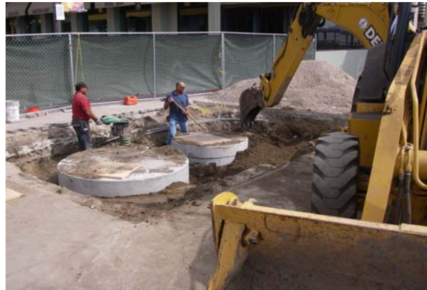
Installation of the two wet wells at the California Street Drain
