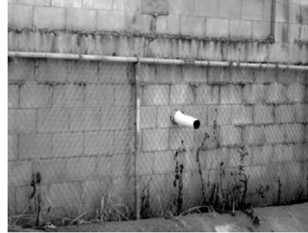
Example of an Illegal Connection
