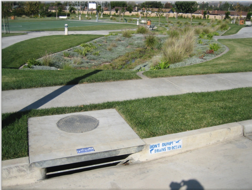
Low Impact Development BMP
