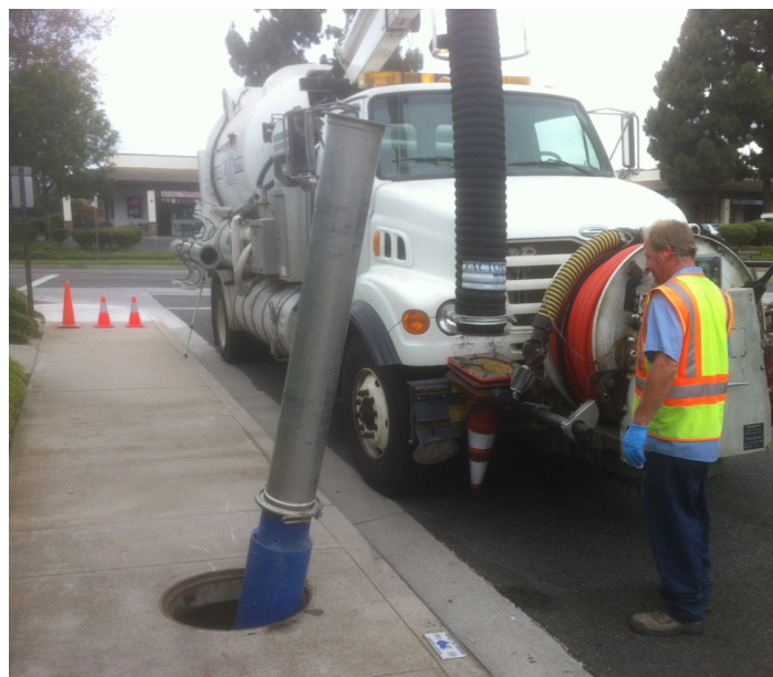
Catch Basin Cleaning Using a Vacuum Truck
