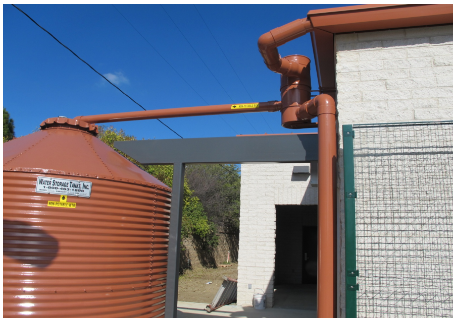
Cistern installation at a cemetery
