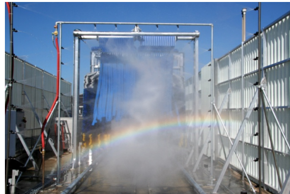
Thousand Oaks’ car wash facility drains to wastewater treatment plant
