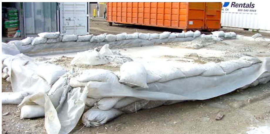
Concrete washout at construction site
