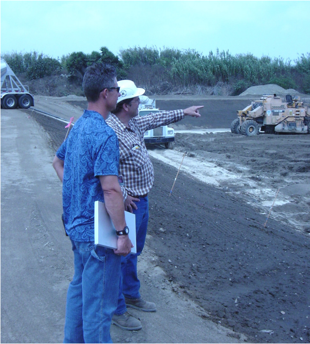
Stormwater inspection at construction site
