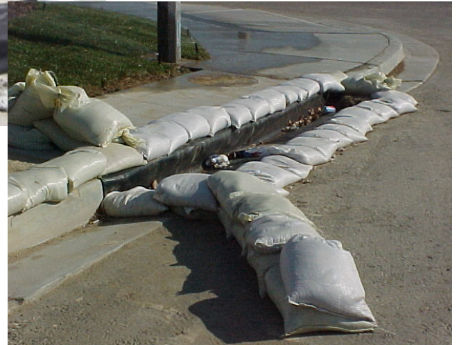
Catch basin protection
