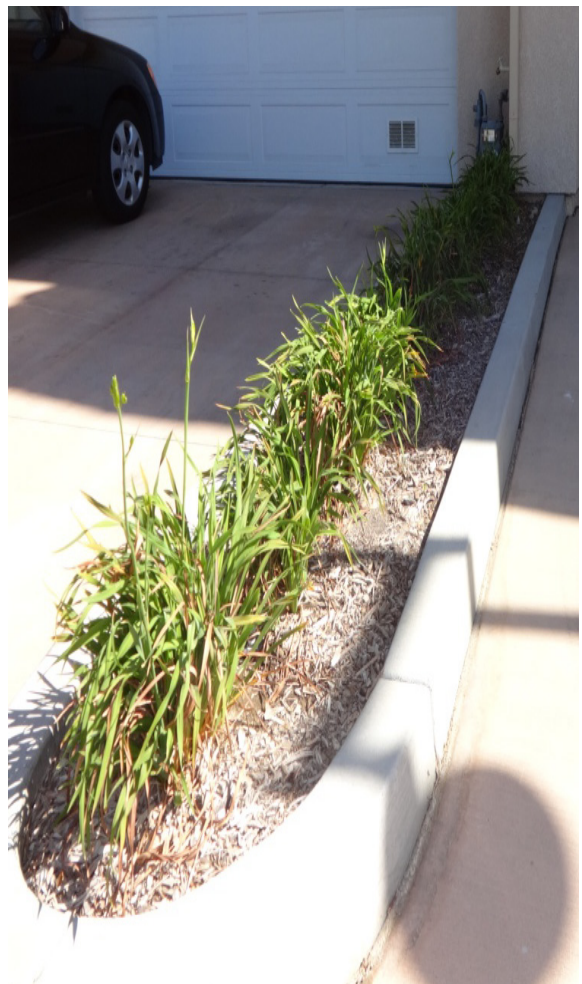
Diverted down spout from rain gutters
