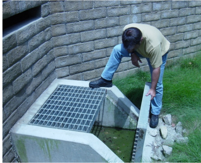
Post-Construction BMP inspection
