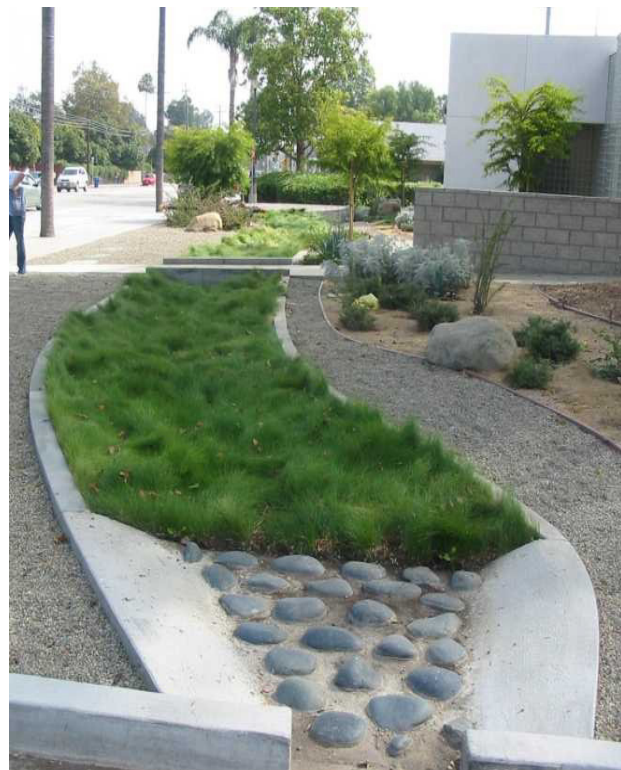
A curb cut leading to an LID feature
