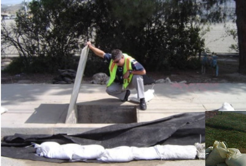
Inspection of catch basin BMPs
