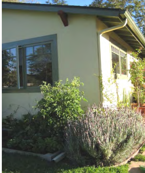
Diverted Roof Runoff City of Santa Barbara
