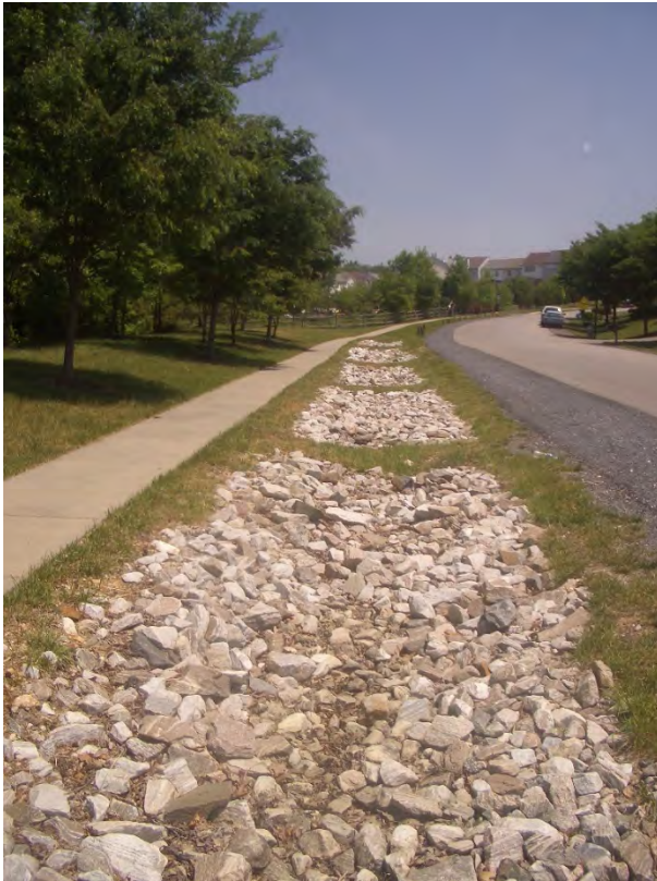
Rural Highway Infiltration Trench
