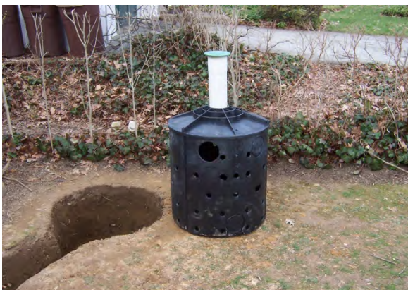
Drywell installation
