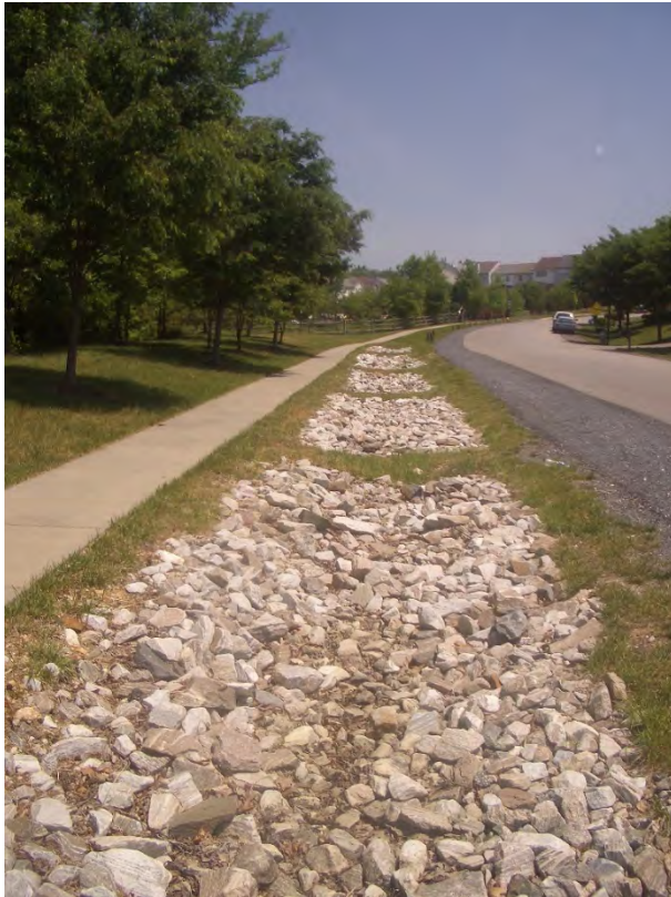
Rural Highway Infiltration Trench
