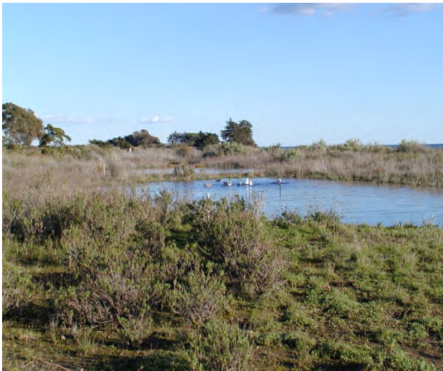
Wet Detention Basin
