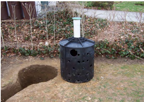
Drywell installation
