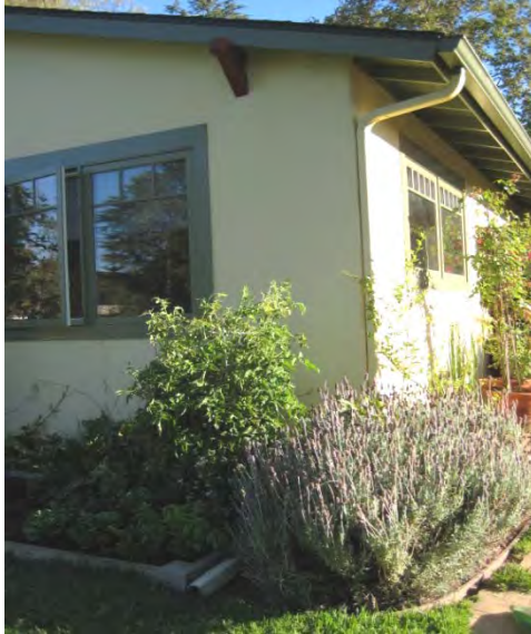
Diverted Roof Runoff City of Santa Barbara
