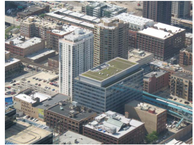
Green Roof Example
