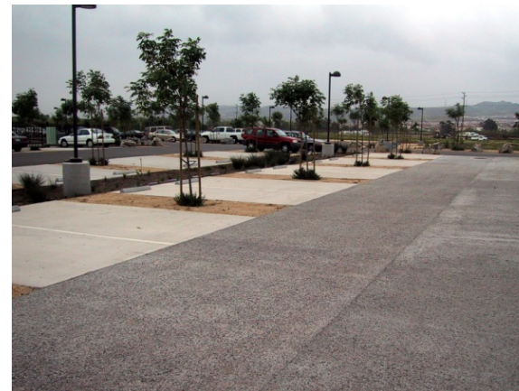
Permeable pavement application
