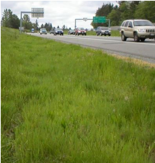
Vegetated filter strip captures runoff from freeway
