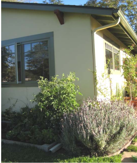
Diverted Roof Runoff City of Santa Barbara
