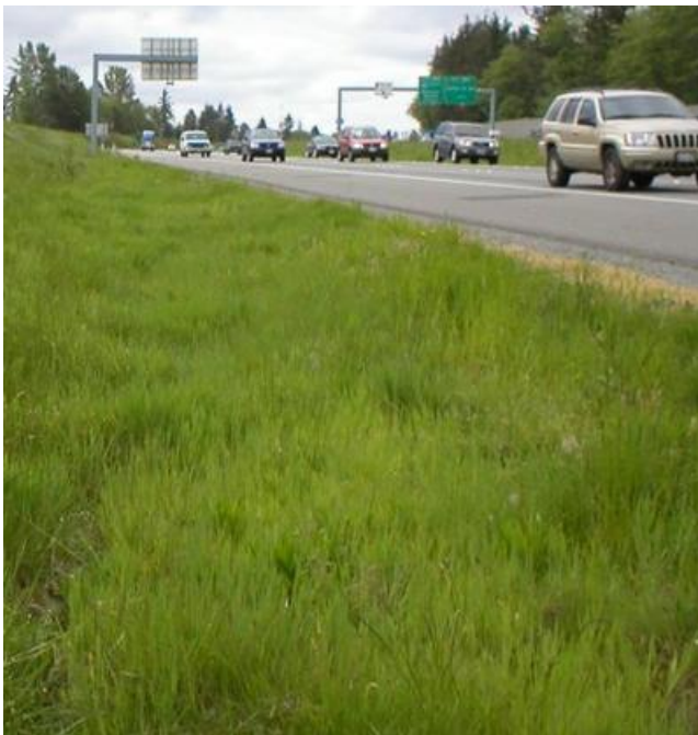
Vegetated filter strip captures runoff from freeway
