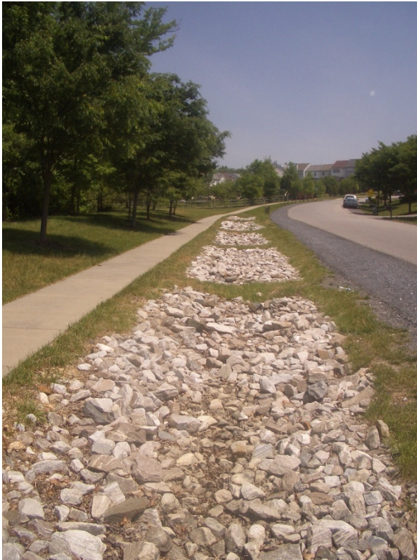
Rural Highway Infiltration Trench
