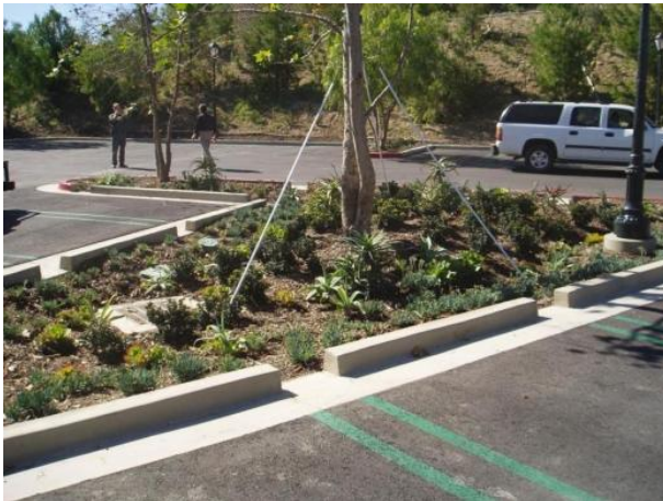
Bioretention in Parking Lots
