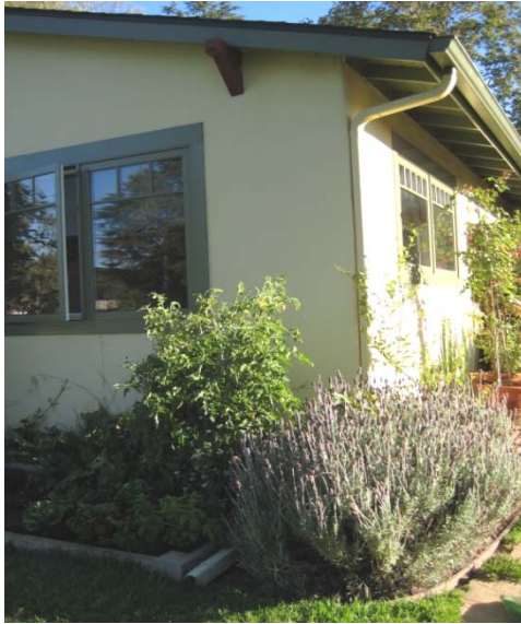
Diverted Roof Runoff City of Santa Barbara
