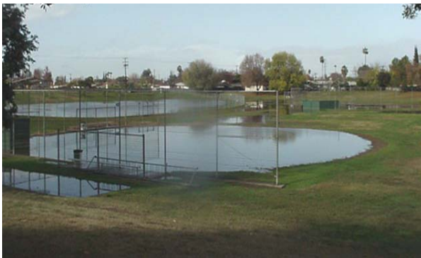
Infiltration Basin in a Fresno, CA Park, Before and After a Rain Event
