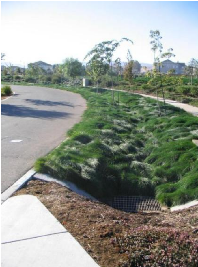
Vegetated swale captures flow from a residential street
