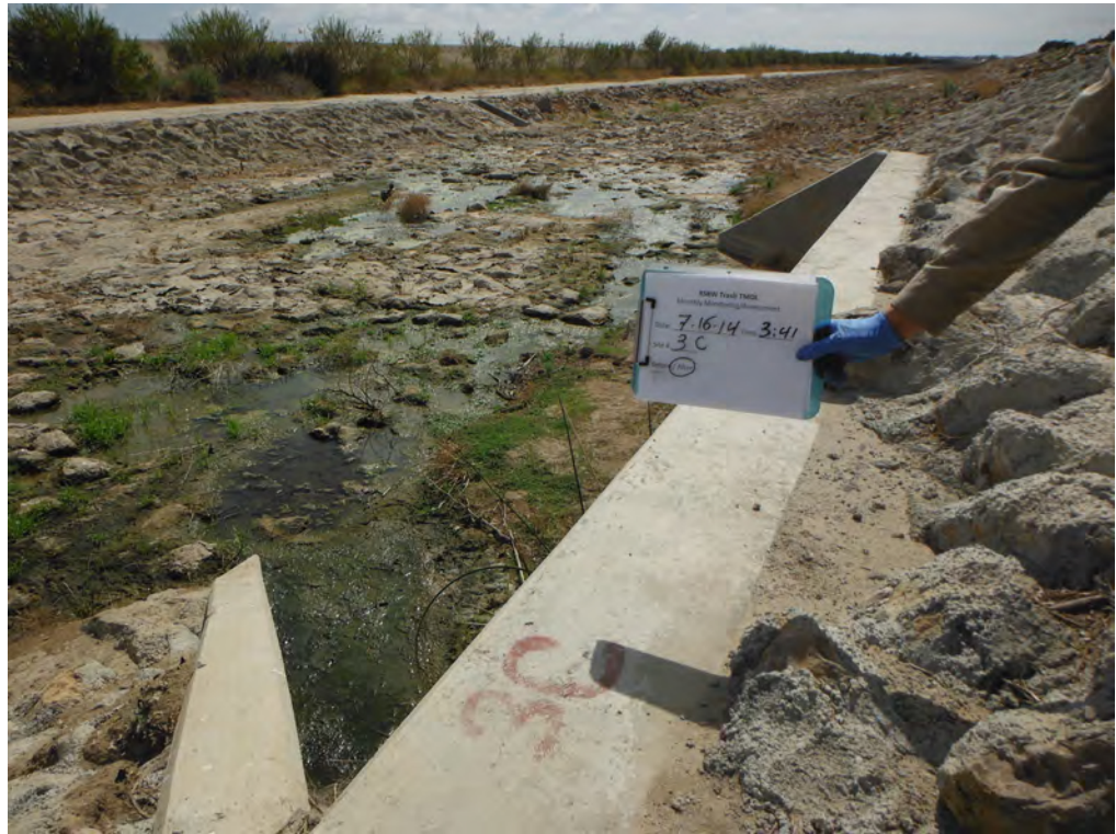
Figure 3-19: Before and After Pictures from a Typical MFAC Event.
