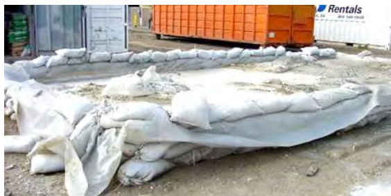
Concrete washout at construction site
