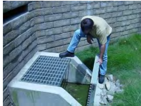
Post-Construction BMP inspection
