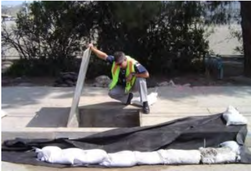
Inspection of catch basin BMPs
