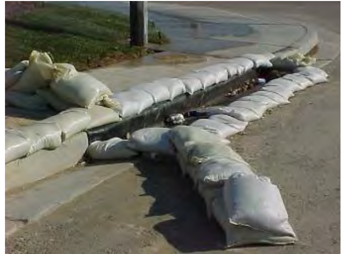
Catch basin protection
