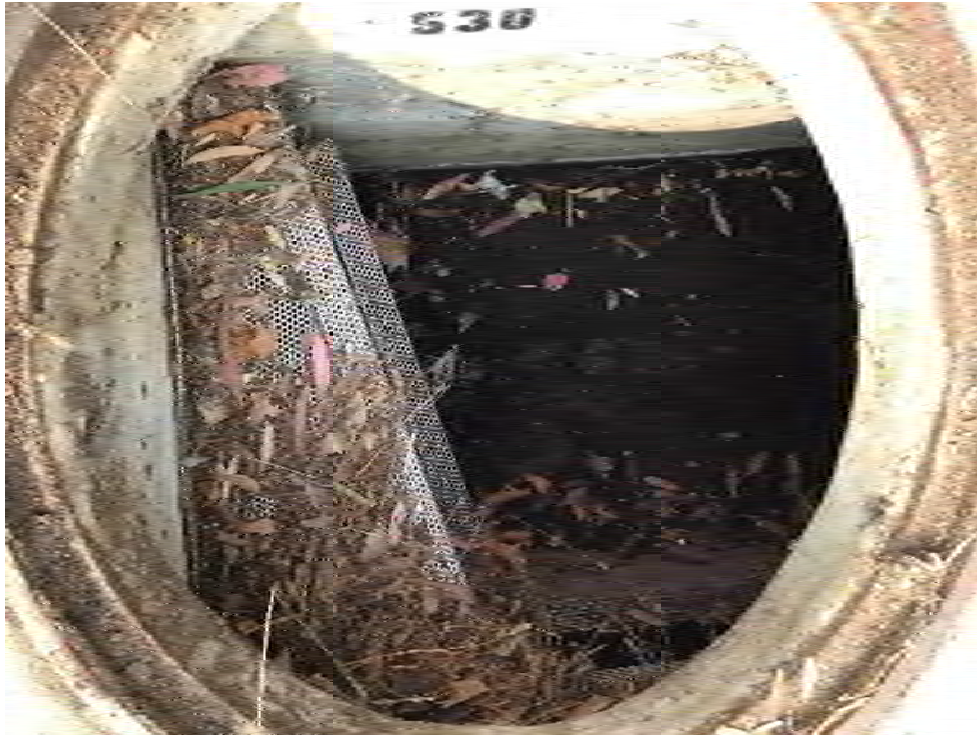
Figure 1: Catch basin prior to cleaning
