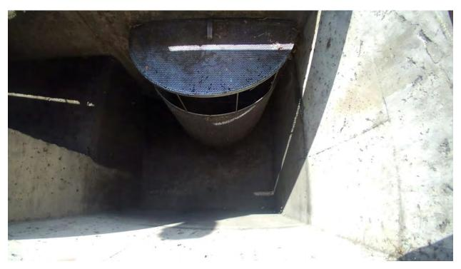
Figure 2: Cleaned catch basin (City of Camarillo catch basin)
