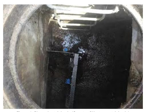
Figure 4: Cleaned catch basin (County of Ventura catch basin)
