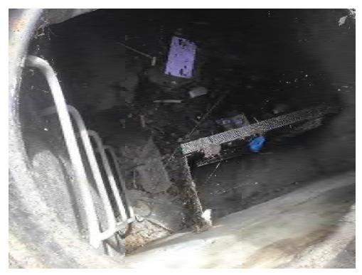
Figure 3: Catch basin prior to cleaning (County of Ventura catch basin)
