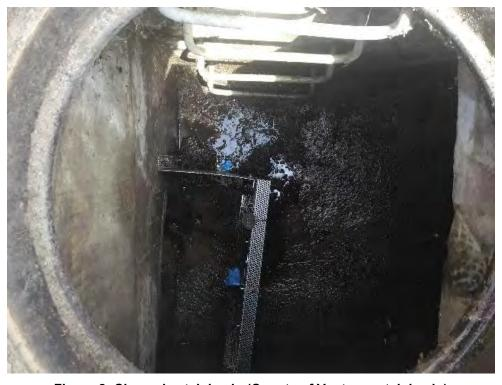
Figure 2: Cleaned catch basin (County of Ventura catch basin)
