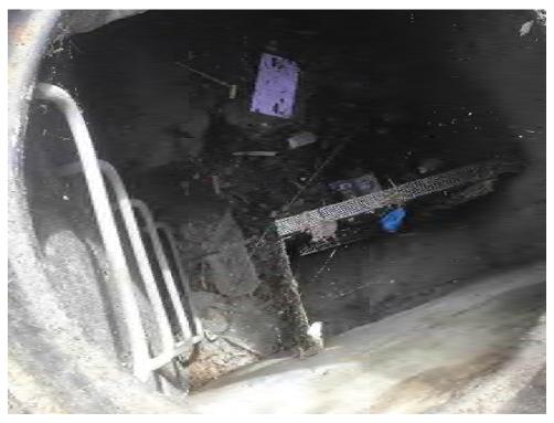
Figure 1: Catch basin prior to cleaning (County of Ventura catch basin)
