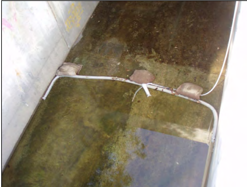
Figure 9-8. Typical Wet-Season, Dry-Weather Sampling Configuration
