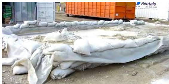
Concrete washout at construction site
