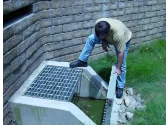
Post-Construction BMP inspection
