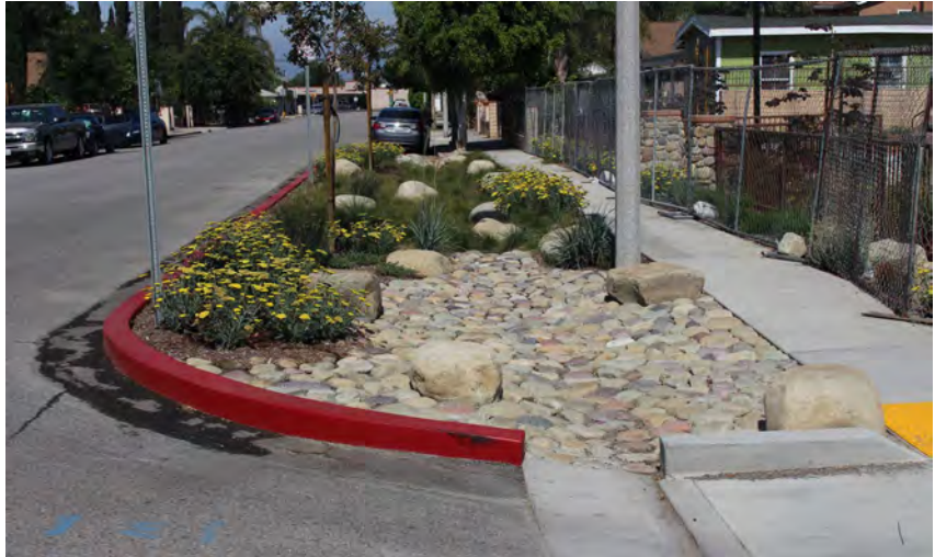
Low Impact Development infiltration BMP
