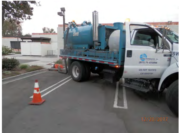
Catch Basin Cleaning Using a Vacuum Truck
