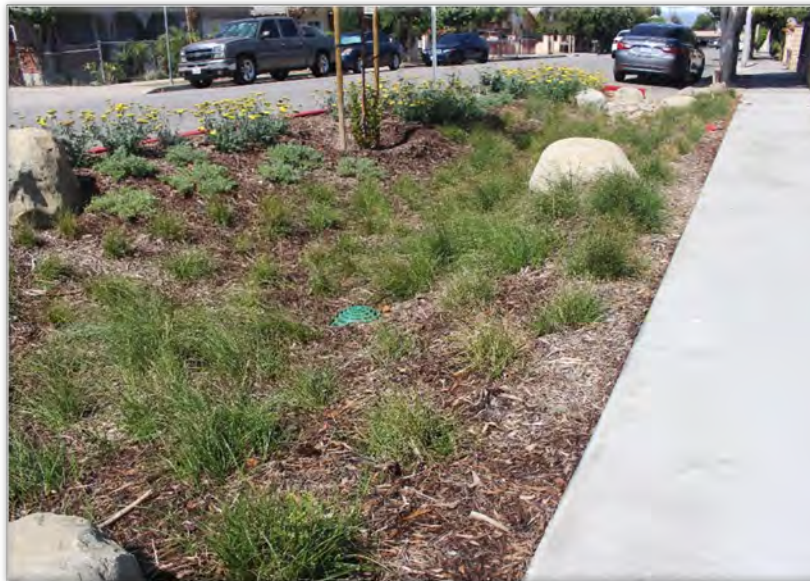
Low Impact Development BMP
