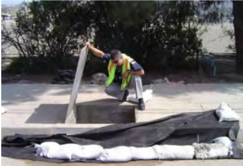
Inspection of catch basin BMPs
