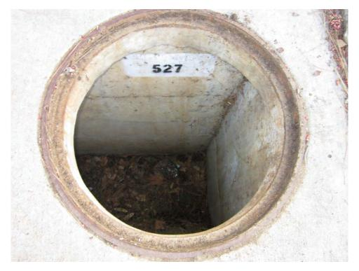
Figure 1: Catch basin prior to cleaning
