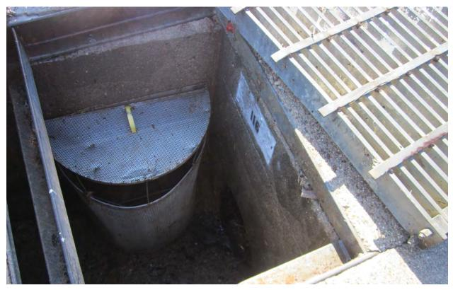
Figure 4: Cleaned catch basin (County of Ventura catch basin)
