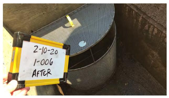
Figure 2: Cleaned catch basin (County of Ventura catch basin)
