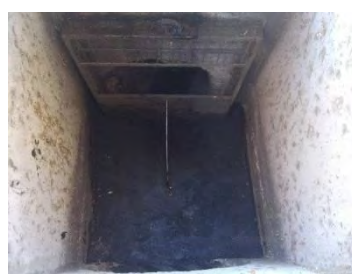
Full Capture Device Cleanout
