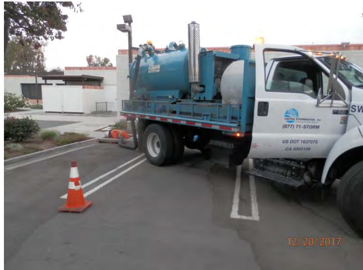
Catch Basin Cleaning Using a Vacuum Truck
