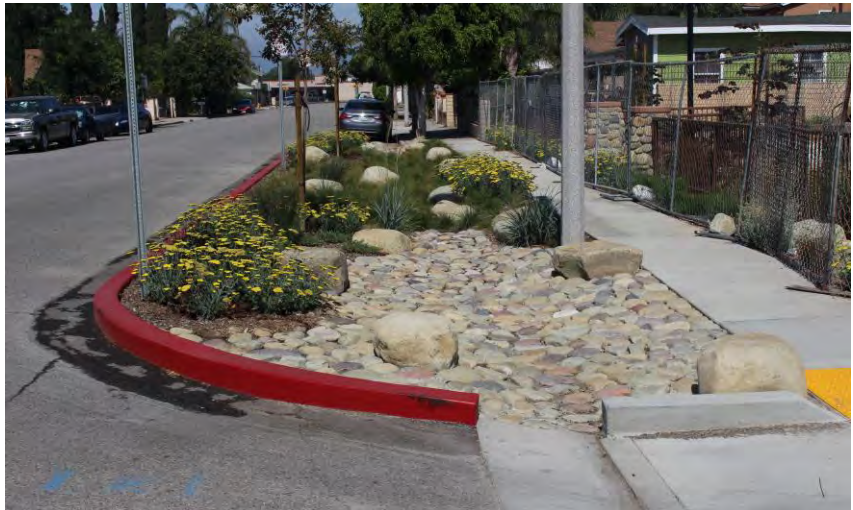
Low Impact Development infiltration BMP
