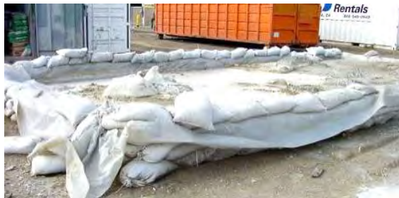
Concrete washout at construction site
