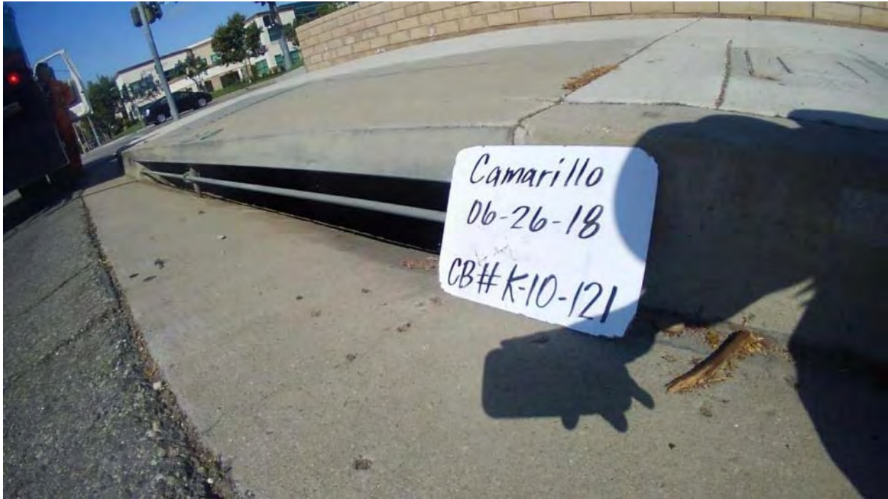
Figure 1. Catch Basin # K-10-121 view from street in June, 2018
