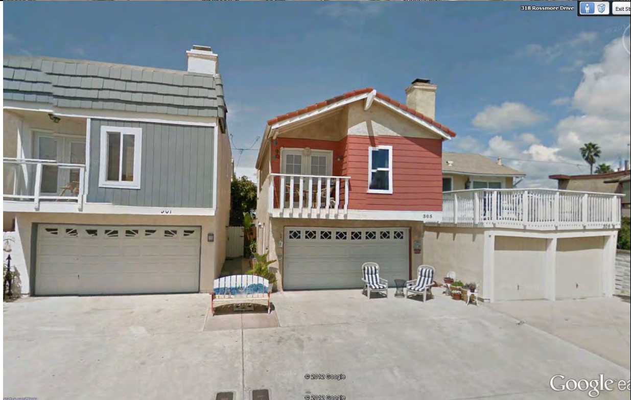
SILVER STRAND, CA - Rossmore Drive, 301-309: 3 ft side yard setbacks, 5 ft rear setbacks, 20 ft paved front yard setbacks. Few or no gutters or downspouts, little or no landscaping to direct water to.
