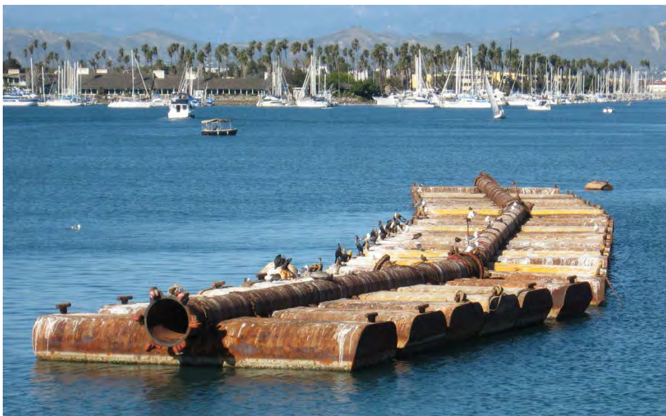
Fig. 1. Birds roosting on pontoon structure used for harbor dredging.
