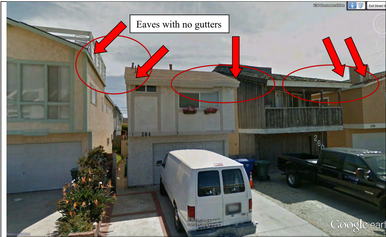
Rossmore Drive 272-256 (About 10% of homes in this area have gutters or downspouts)
