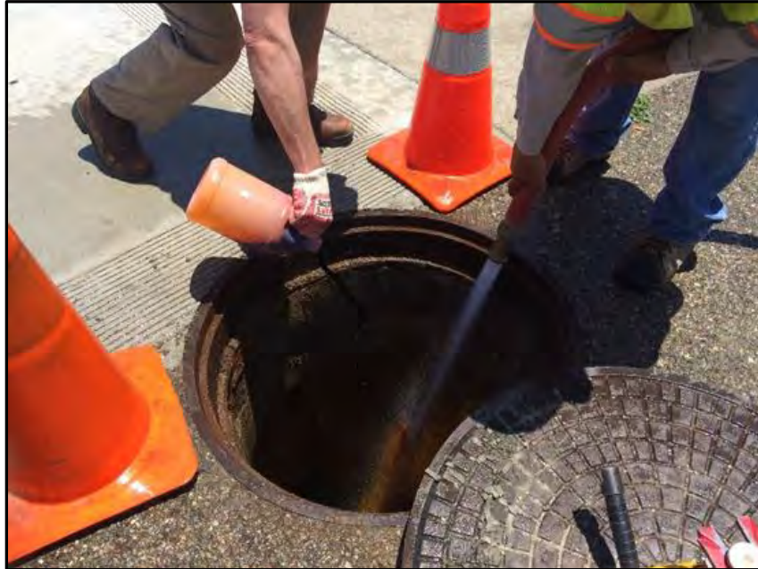
Location #1 Manhole (Provided by the County)
