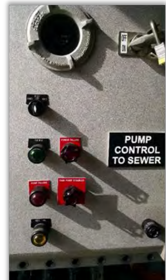
Pump Controls (Provided by the County)
