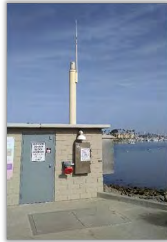
Stand pipe rain gage on roof of pump house (Provided by the County)
