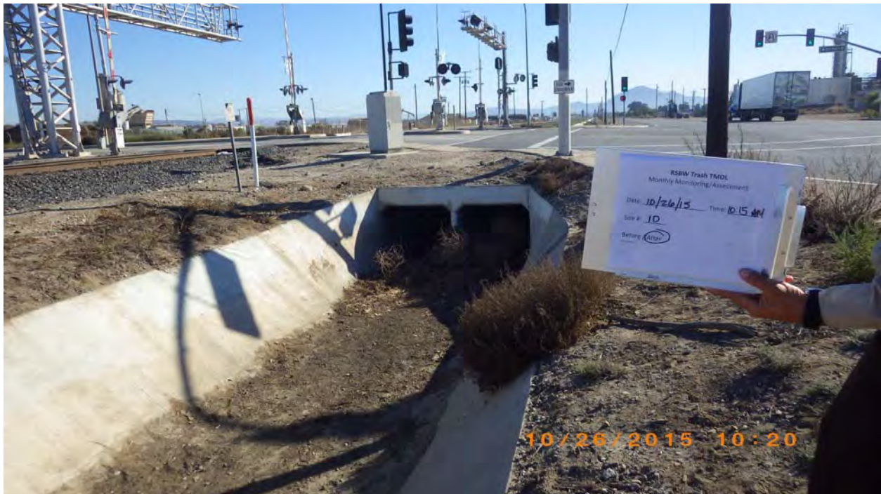
Figure 10. Site 10 before a MFAC Event in October, 2015
