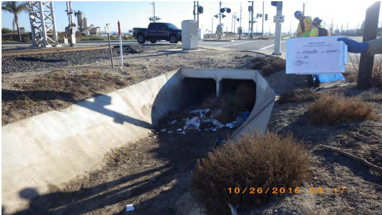
Figure 9. Site 10 before a MFAC Event in October, 2015
