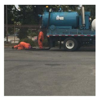
Catch Basin Cleaning Using a Vacuum Truck
