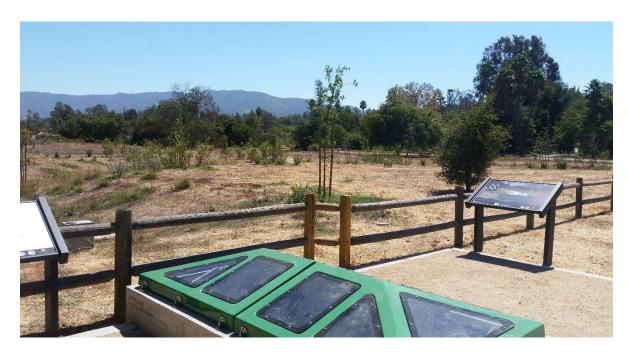
3. El Rio Retrofit for Groundwater Recharge. Construction was completed in March 2016. The project captures 100% nuisance flows and the first flush stormwater discharges from 46 acres of residential community of El Rio for infiltration and groundwater recharge. Total project cost is \$1.3M.
