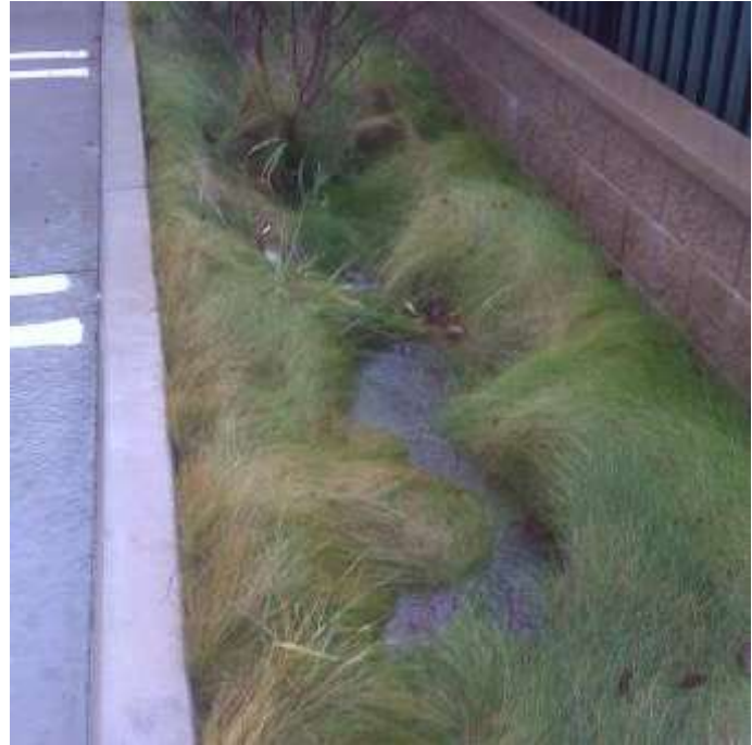
Low Impact Development infiltration BMP
