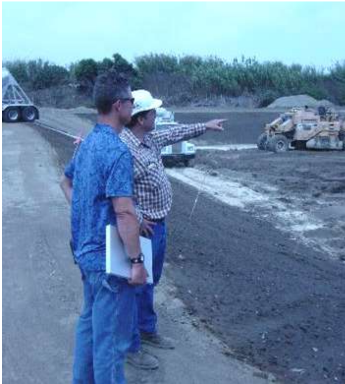
Stormwater inspection at construction site
