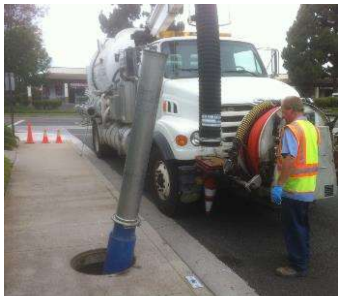
Catch Basin Cleaning Using a Vacuum Truck
