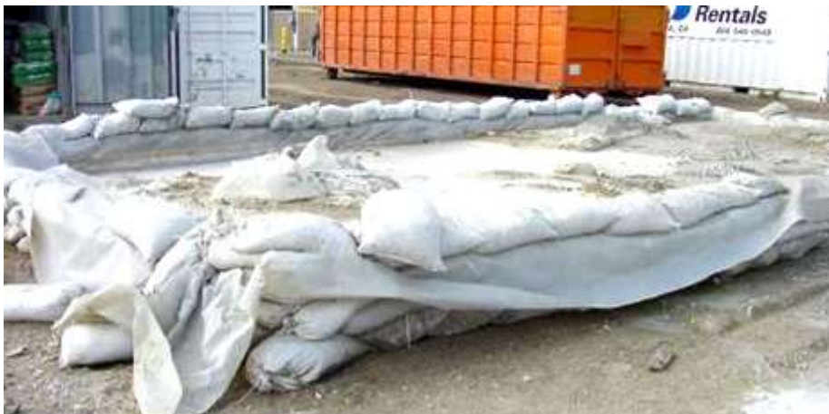
Concrete washout at construction site
