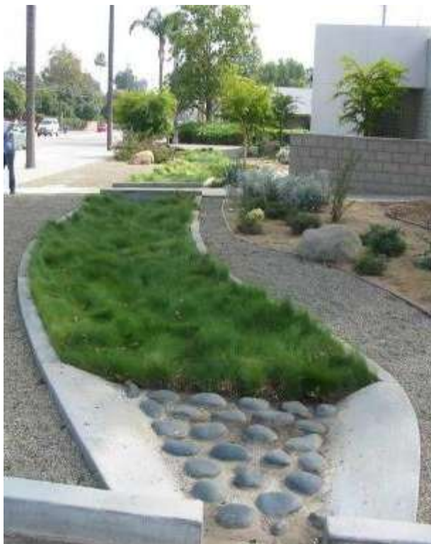
A curb cut leading to an LID feature
