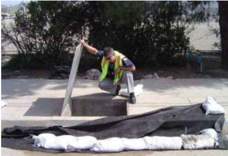
Inspection of catch basin BMPs
