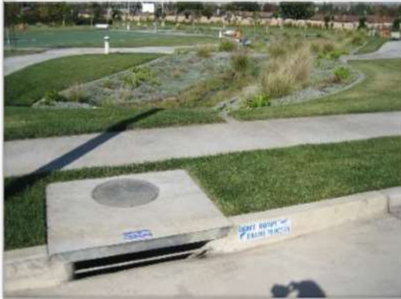
Low Impact Development BMP
