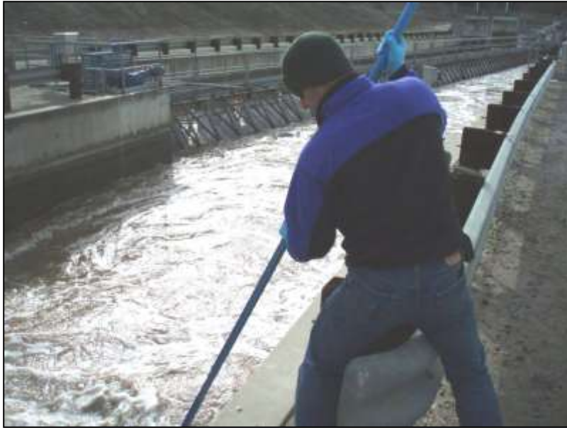
Figure 9-7. Grab Sampling Using Extended-Reach Swing Sampler
