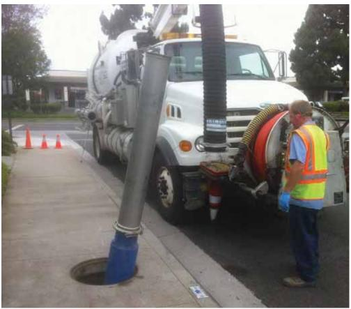
Catch Basin Cleaning Using a Vacuum Truck
