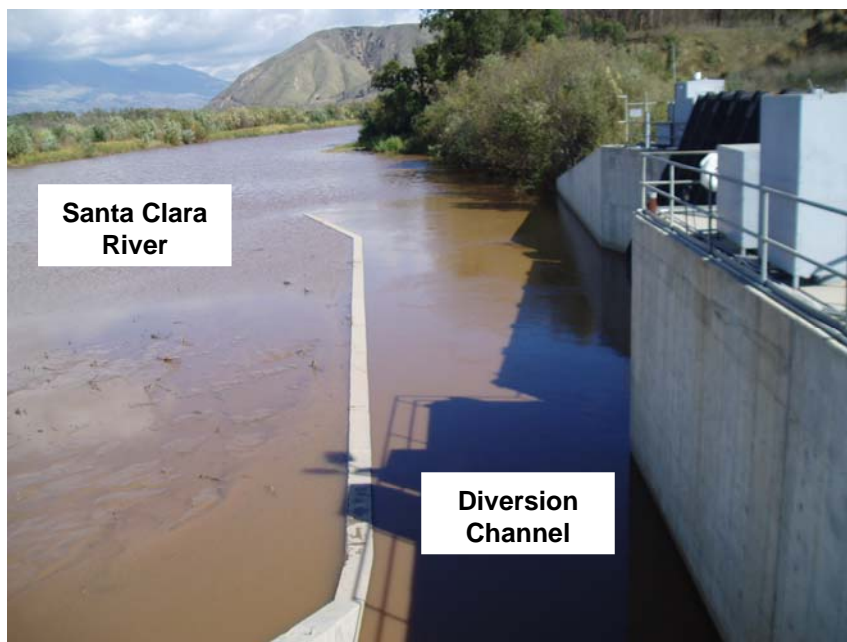
Figure 10: ME-SCR Freeman Diversion Dam (Facing Upstream)
