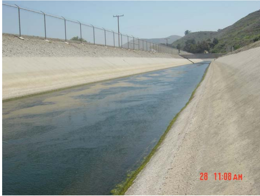
Figure 20: Infiltration Channel (Facing Upstream)
