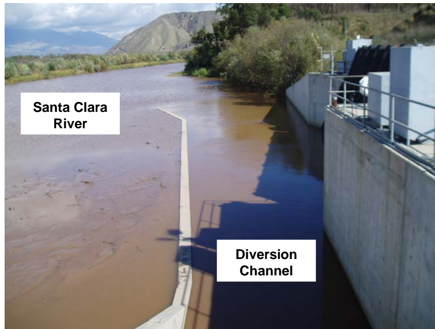
Figure 17: ME-SCR Freeman Diversion Dam (Facing Upstream)
