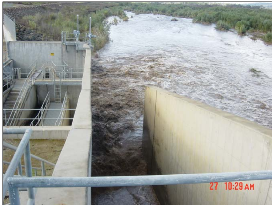
Figure 19: River Diversion Gate (Facing Downstream)
