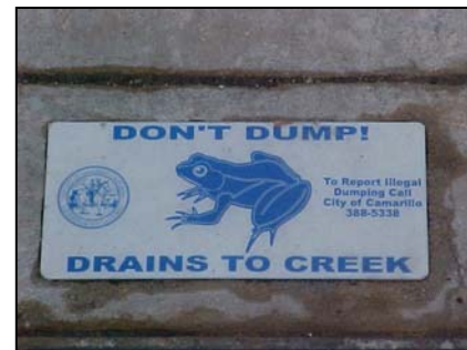
Example of Storm Drain Curb Marker
