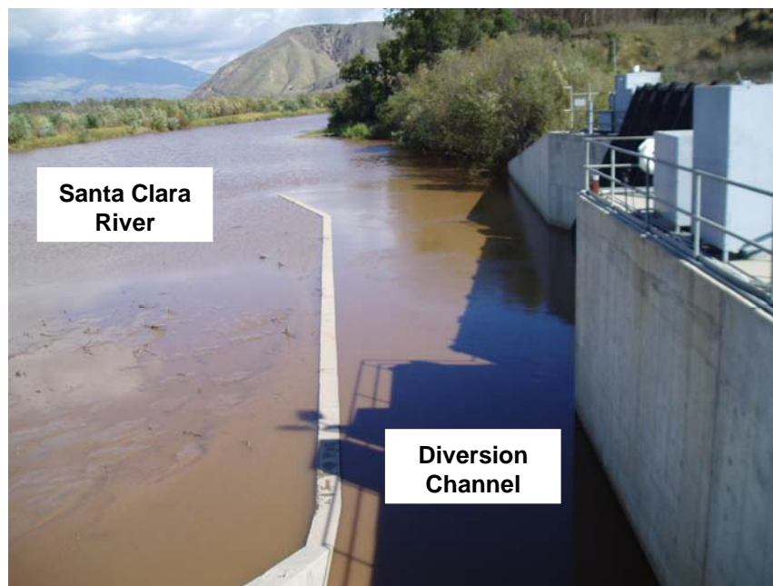
Figure 9-29: ME-SCR Diversion Dam (Facing Upstream)
