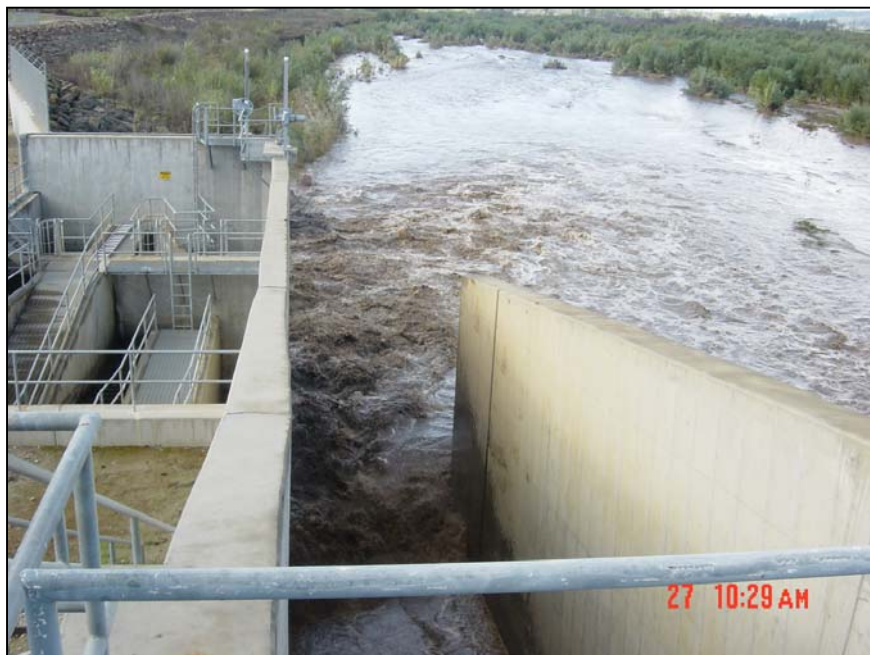
Figure 9-31: River Diversion Gate (Facing Downstream)
