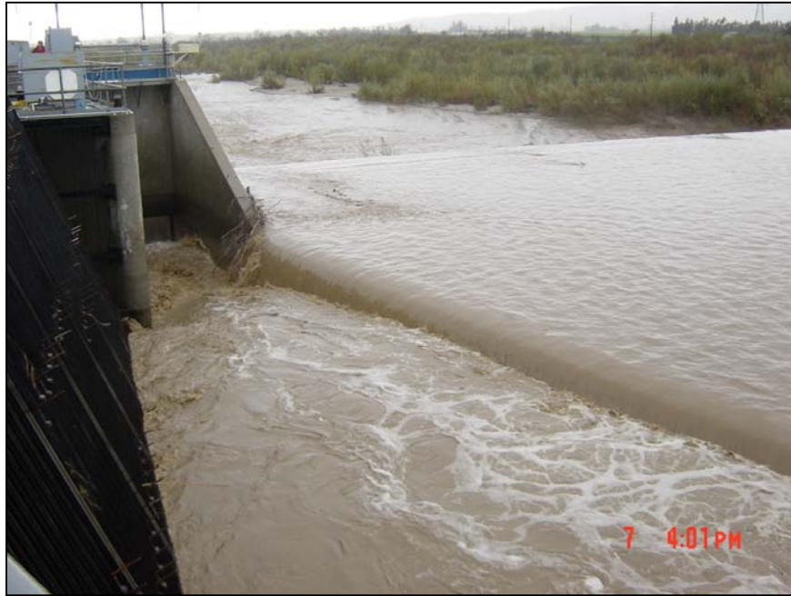
Figure 9-30: ME-SCR Diversion Dam (Facing Downstream)
