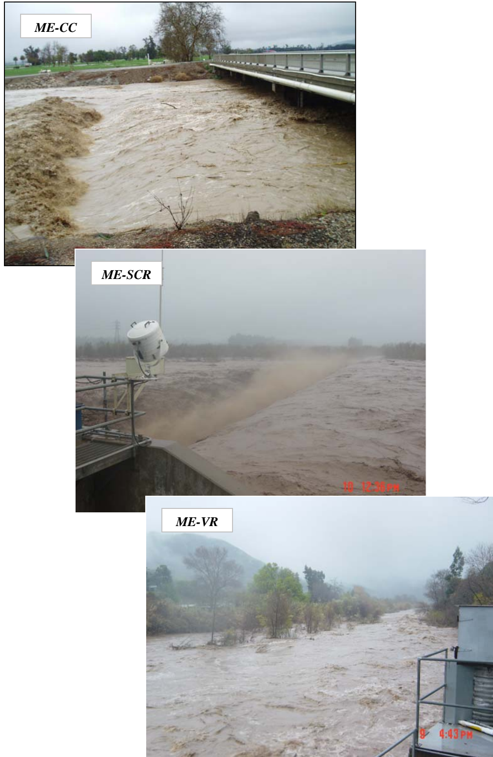
Figure 9-18: Mass Emission Station Photos: ME-CC (Calleguas Creek), ME-SCR (Santa Clara River), and ME-VR (Ventura River) during high flows in early January 2005 (Event 4)
