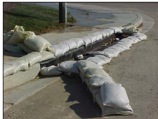
Example of Inlet Protection
