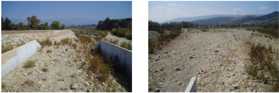
Station 6 - Ventura River at Santa Ana Rd. Dry
