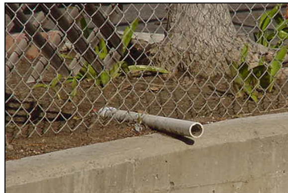
Example of an Illegal Connection
